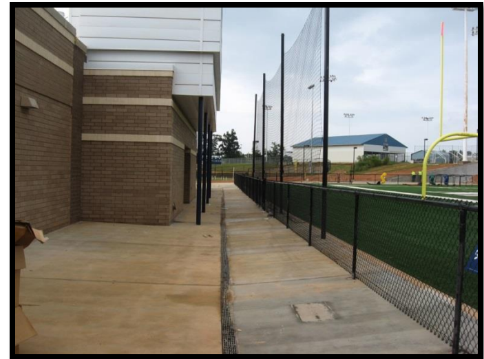
Field side face of Field House
