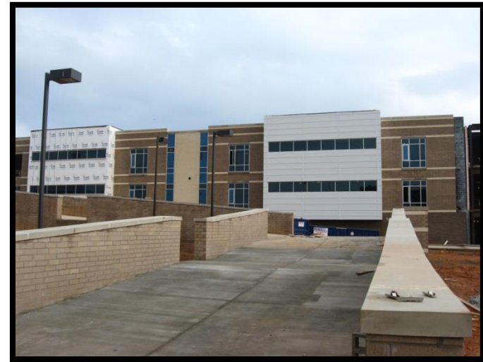
Two Story Classroom Bldg. from Field House
