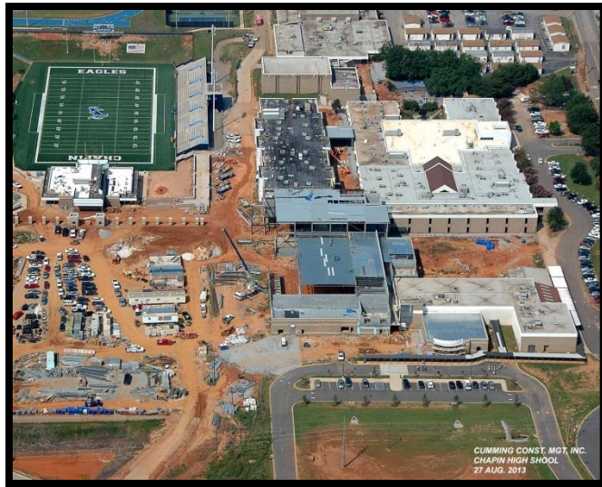
Site Aerial along Columbia Avenue
