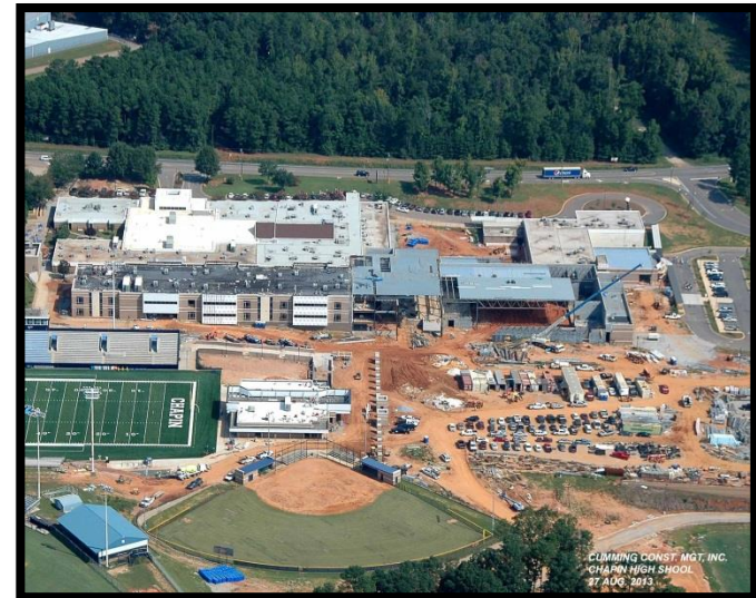
Site Aerial towards Columbia Avenue
