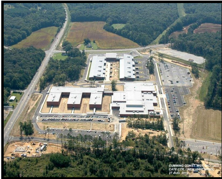
Site Aerial towards CATE
