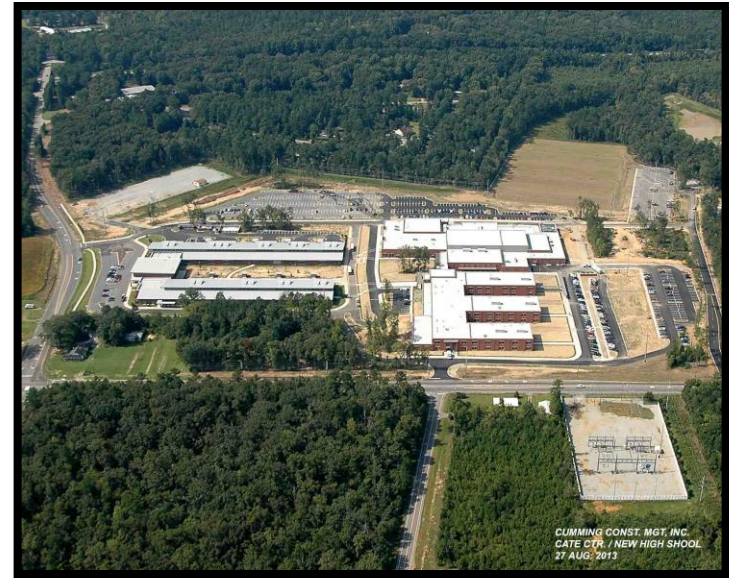
Site Aerial from Broad River Road
