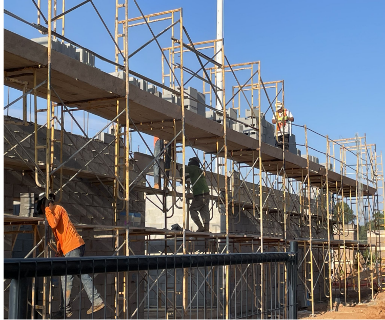
Masonry Began July 24
