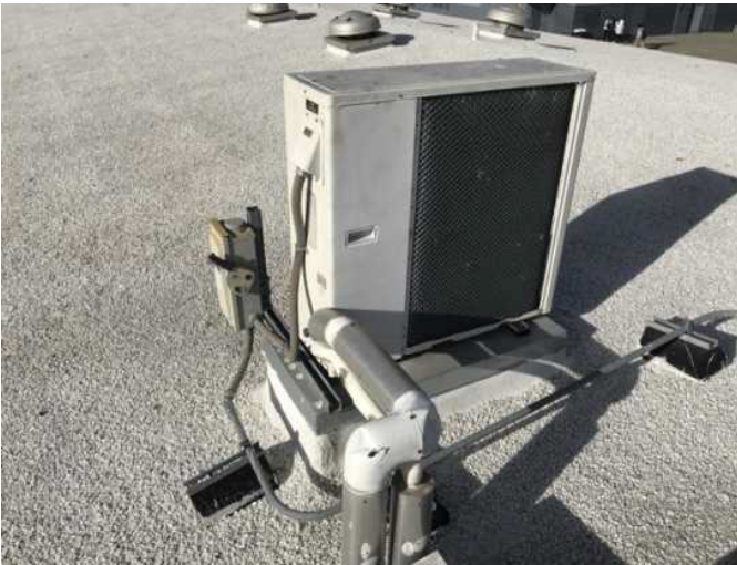
7 - SPLIT SYSTEM DUCTLESS CONDENSING UNIT
