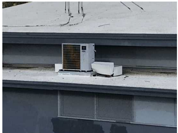
6 - SPLIT SYSTEM DUCTLESS CONDENSING UNIT
