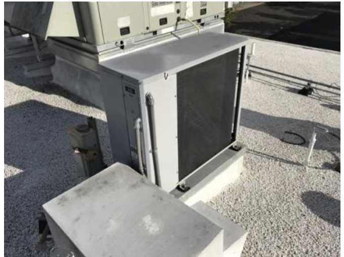
8 - SPLIT SYSTEM DUCTLESS CONDENSING UNIT
