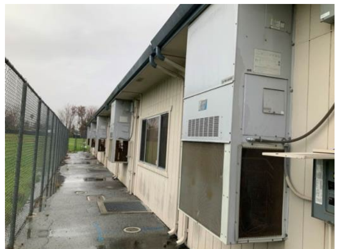
6 - PACKAGED UNITS AND ELECTRICAL PANEL
