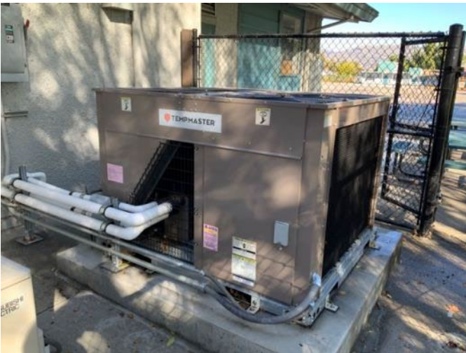
9 – CONDENSING UNIT/HEAT PUMP
