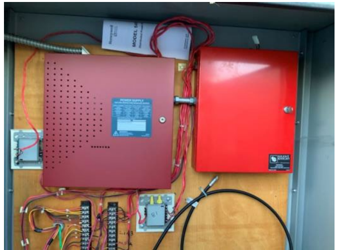
10 - FIRE ALARM COMPONENTS
