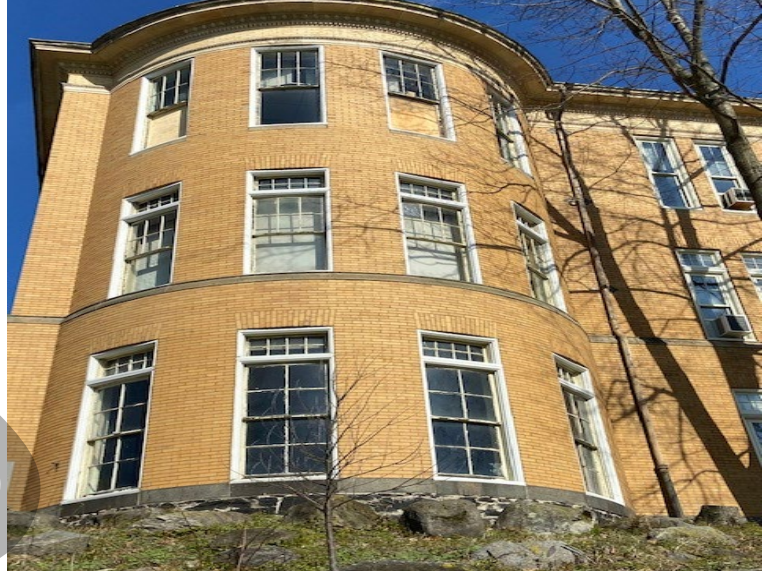
Administration building windows
