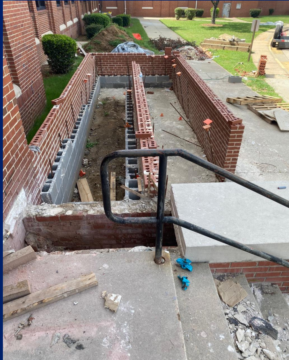
ADA ramp at front entrance
