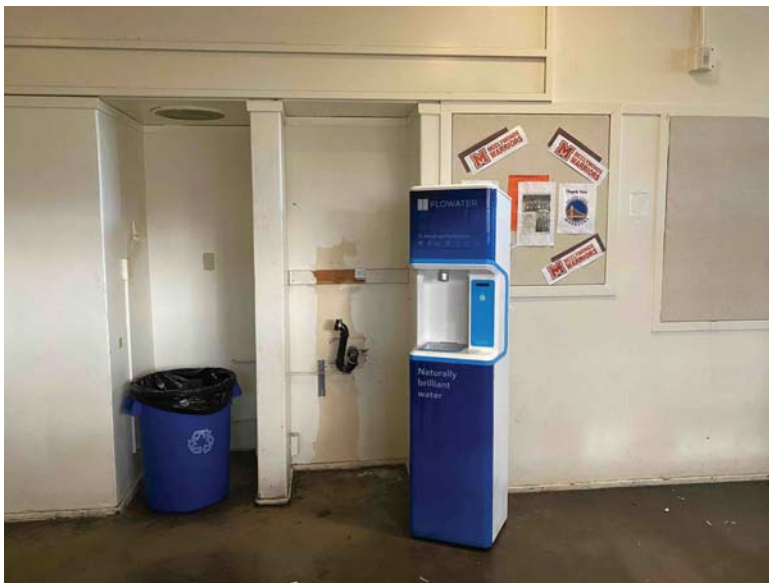
Drinking fountain was replaced with Flowater and is not connected in Wing D Boy's Hallway
