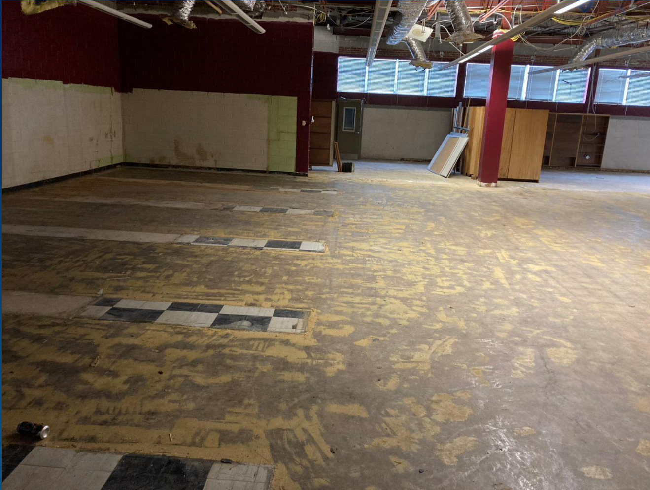
Media Center Demolition
