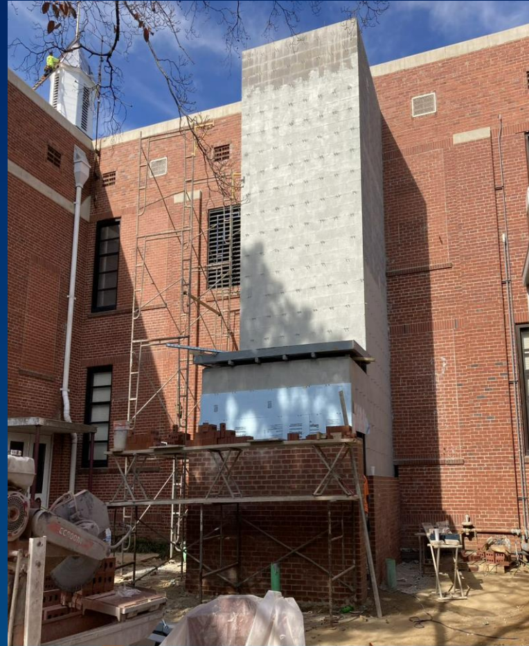
Elevator Shaft
