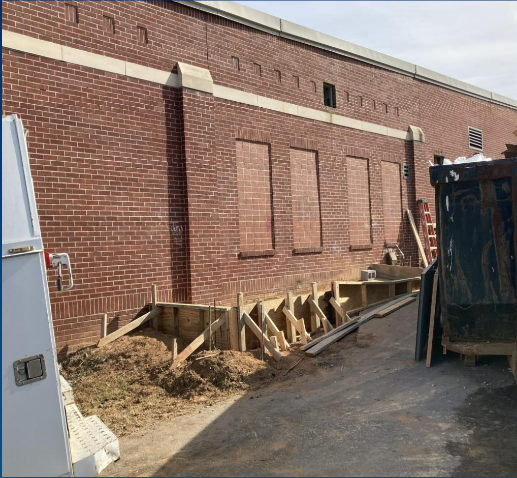
Foundation to Support New HVAC Equipment
