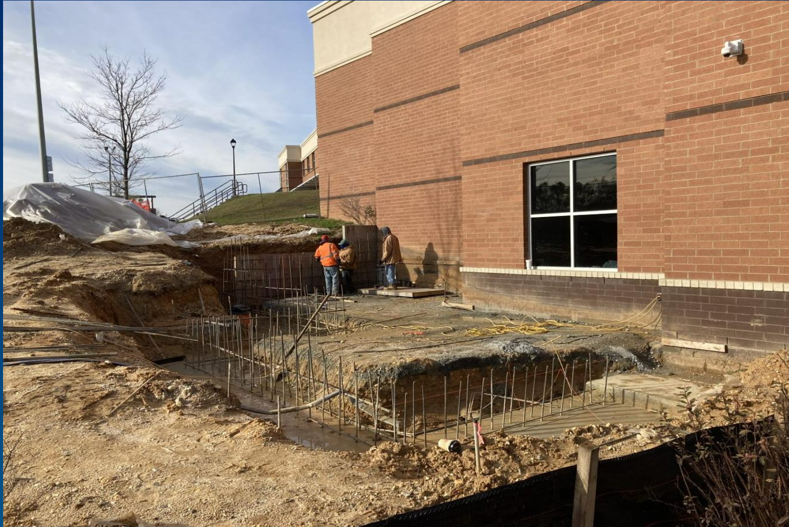
Foundation for Expansion
