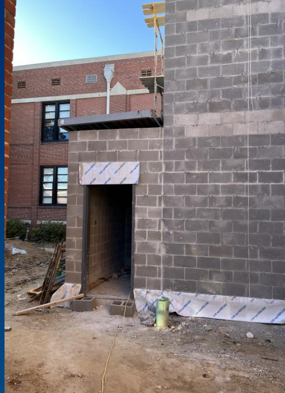
Elevator Shaft
