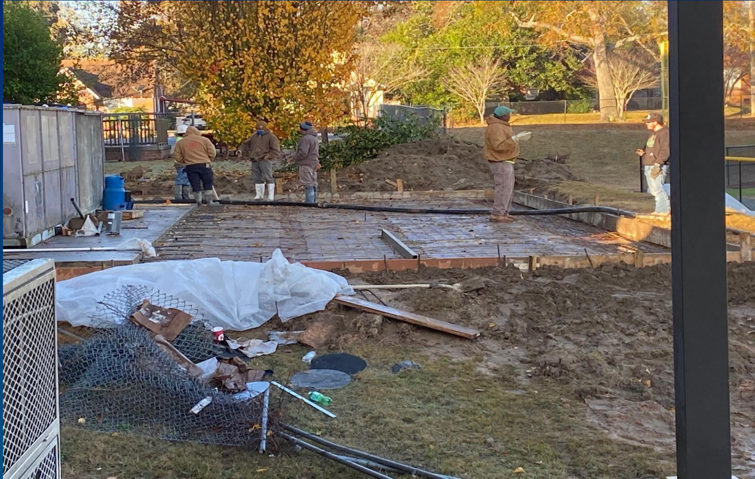
Foundation to Support New HVAC Equipment
