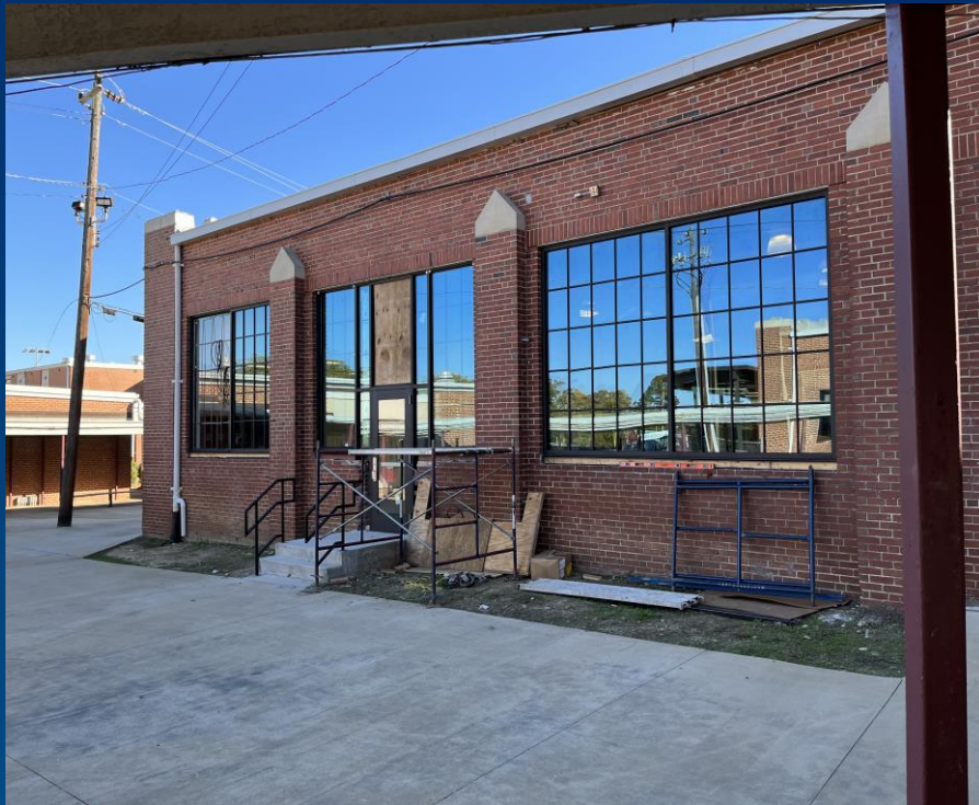
Exterior and Interior of Lab Spaces
