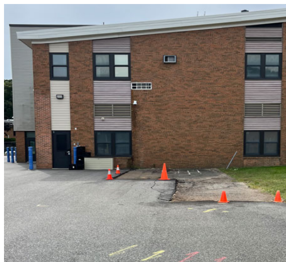
In process – LADSBS Storage containers removed and asphalt repair is pending
