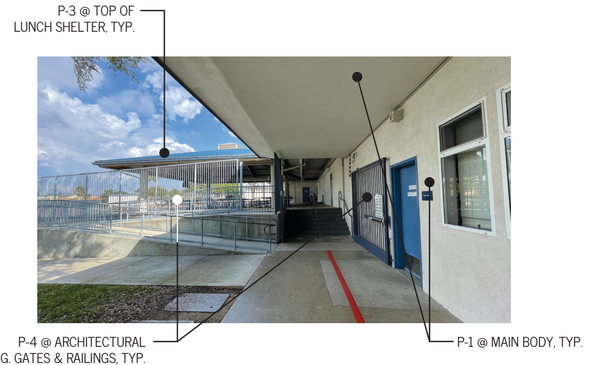
VIEW 7 ADMINISTRATION AND LUNCH SHELTER - TYPICAL AT THIS CONDITION
