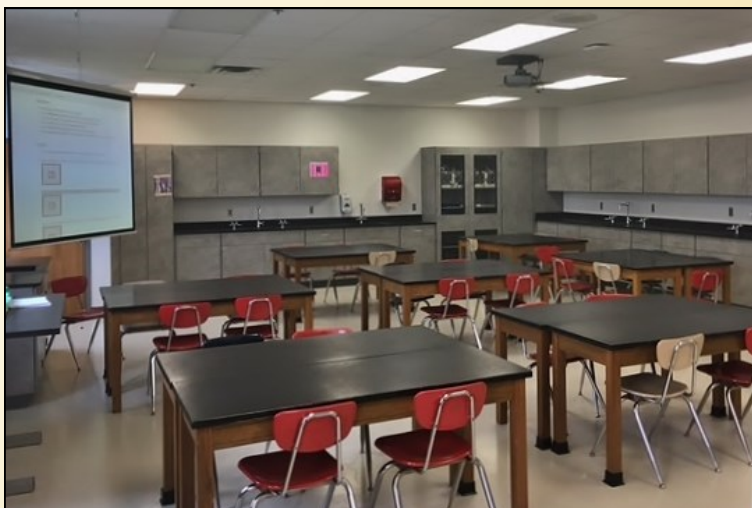
Renovated science lab
