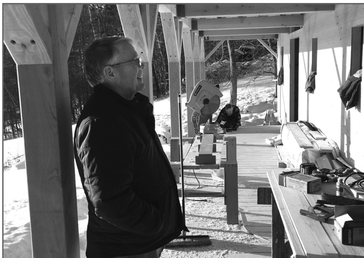
Randy Mudge on a newly constructed porch, which is on the lake side and below the new section of Memorial Hall
