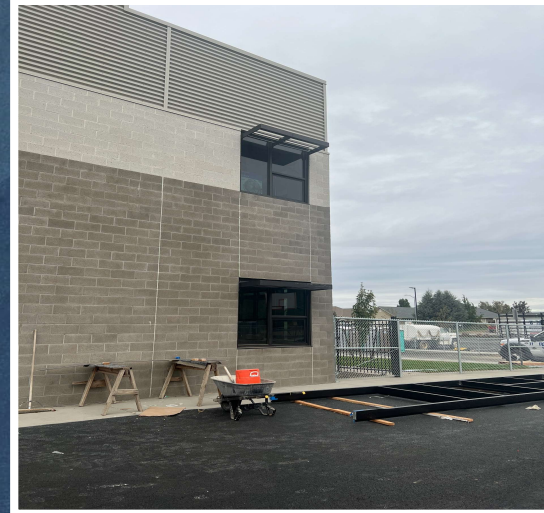
Sunshade Install Ongoing
