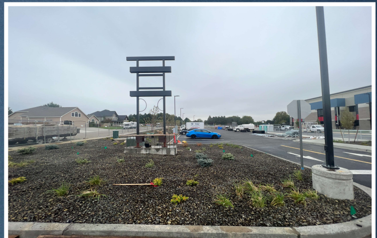
Reader board Install Ongoing
