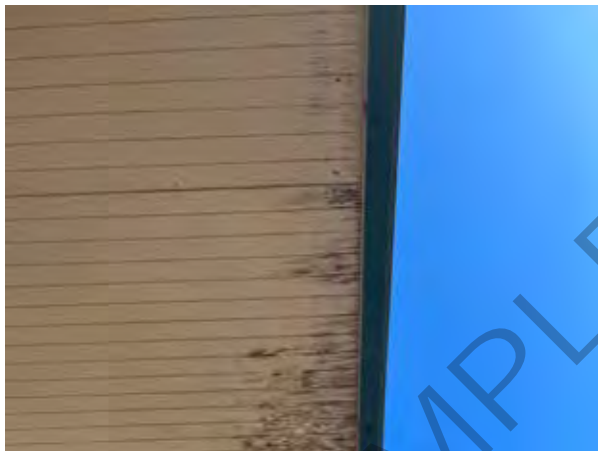
Repair water damage under roof eaves
