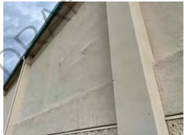
Gymnasium exterior wall water damage
