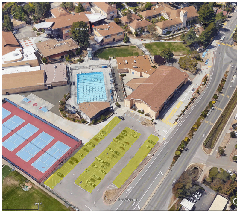
Tam Paring Structures
