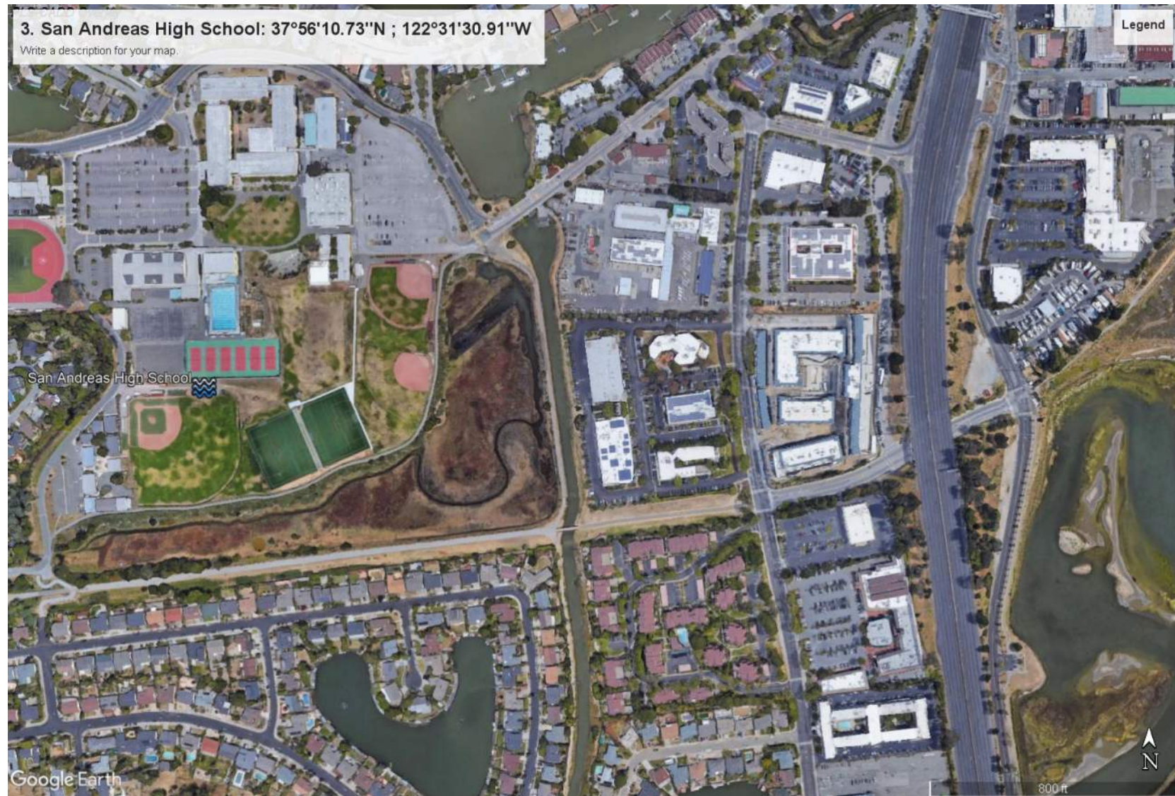
Figure 4: Google Earth near-field image of San Andreas High School locations relative to the shoreline of a Corte Madera Creek tidal channel. Elevation of existing grade at San Andreas High School averages approximately +7 ft. NAVD.
