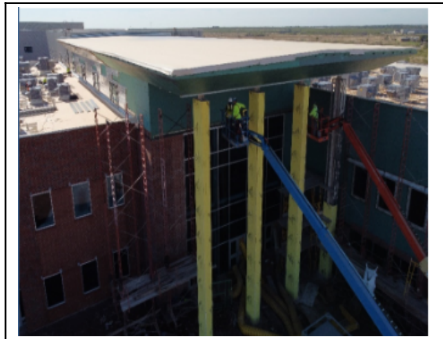
Main entry column framing & sheathing
