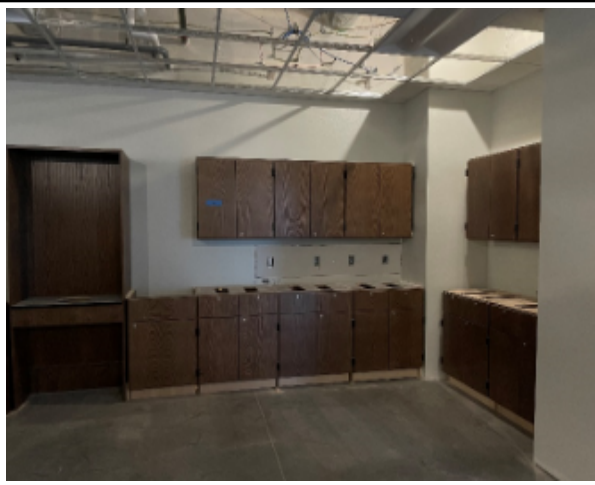
Science lab casework installation
