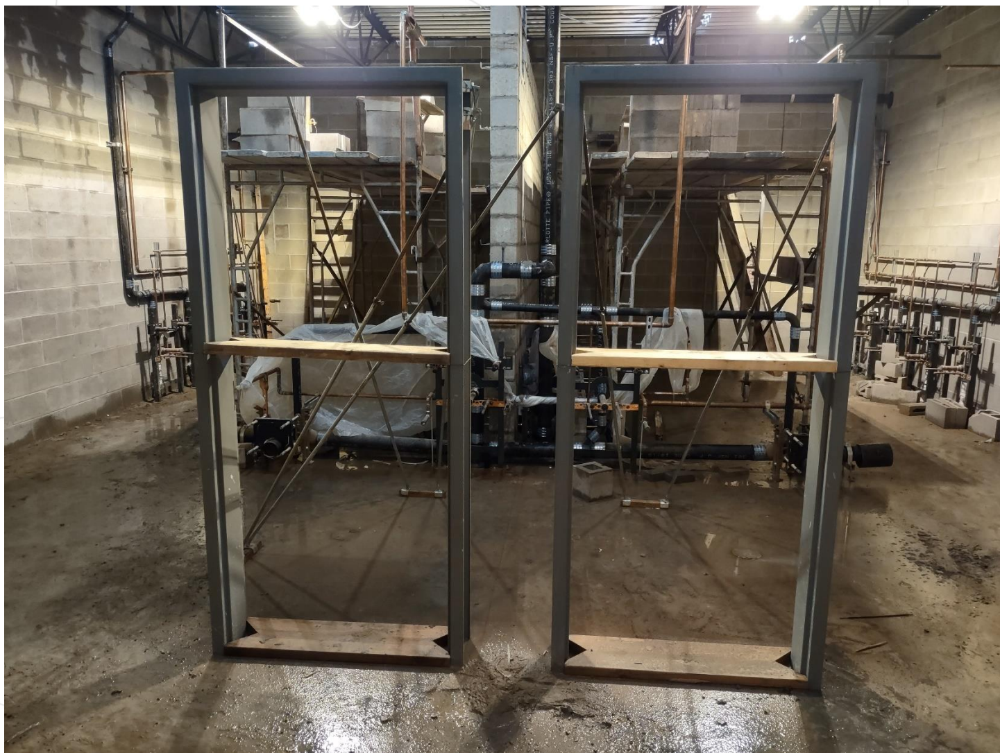
Gang Restroom Rough-ins in Area A Addition
