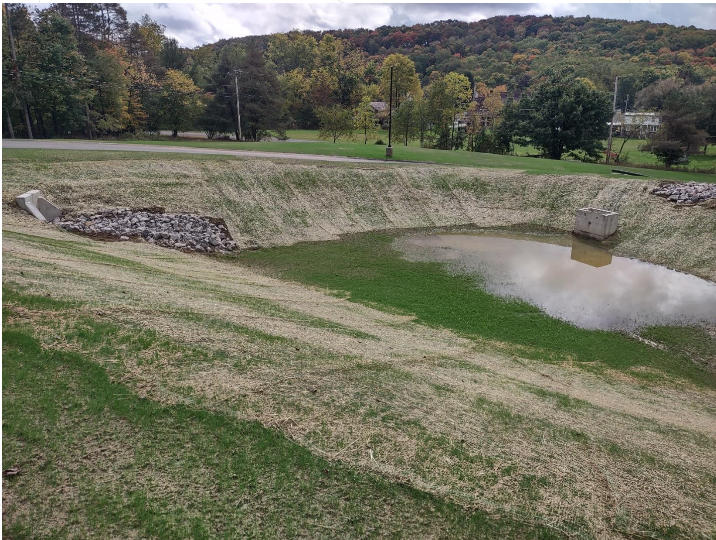
Erosion Control Pond at bottom of hill by Spring Street
