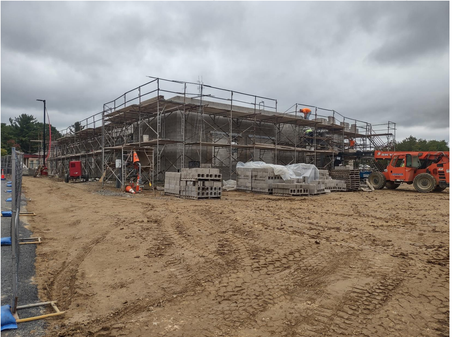
Southeast elevation of new classroom. Masonry is up to Bearing Height
