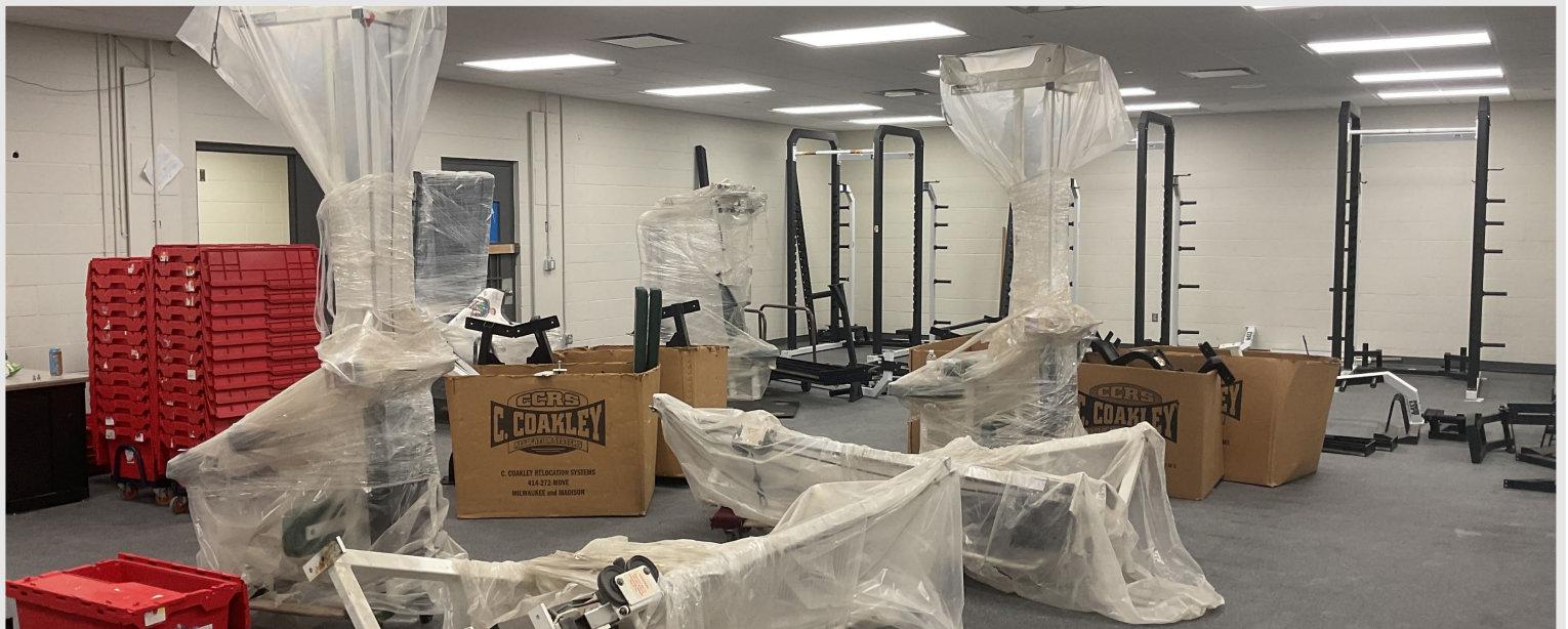
Equipment is being installed in the newly renovated upper-weight room, which received upgraded heating, ventilation, and air conditioning (HVAC), lighting, a new ceiling, and a new, durable rubber floor
