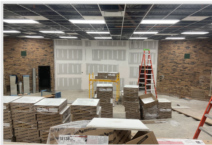
The new wall in the front of the small theater (Theater 300) is ready to be painted, and lights and ceilings are being installed
