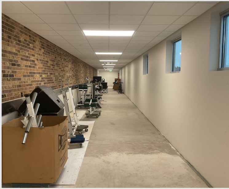
The new second-floor corridor improves traffic flow and accessibility to multiple spaces in the building
