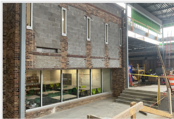
Concrete work is complete in the new commons area, with classrooms overlooking the new space
