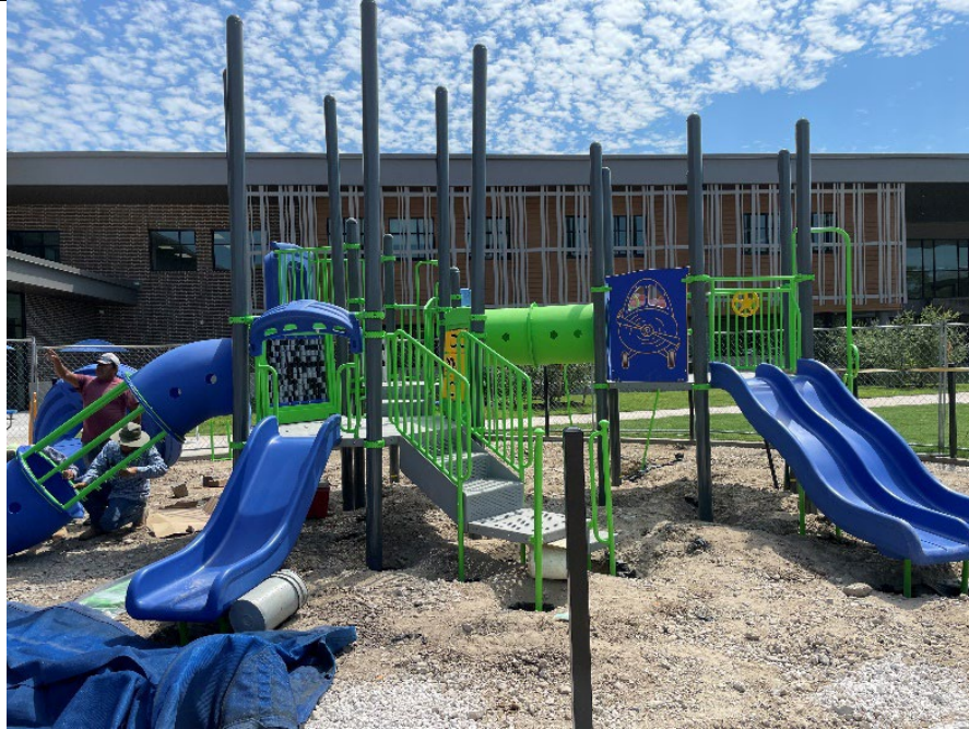
Playground: Progress view of playground equipment installation in the playground Area.
