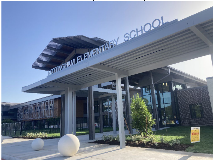
Exterior: View at entrance of school.
