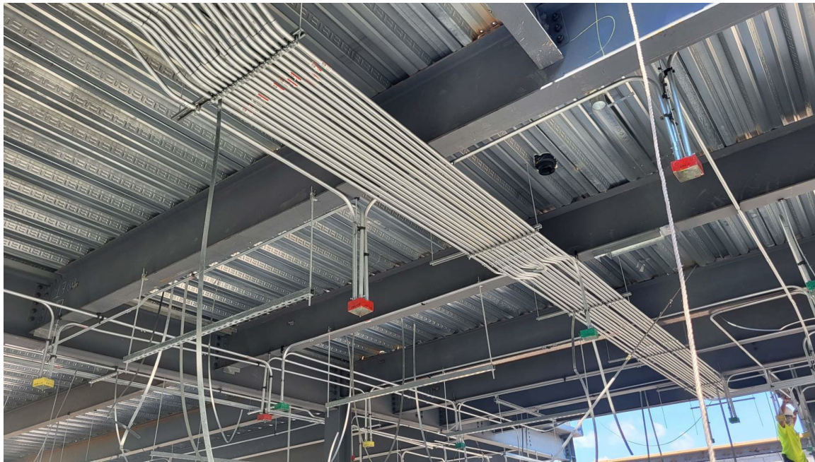
Area F Overhead Electrical and Duct Hangers
