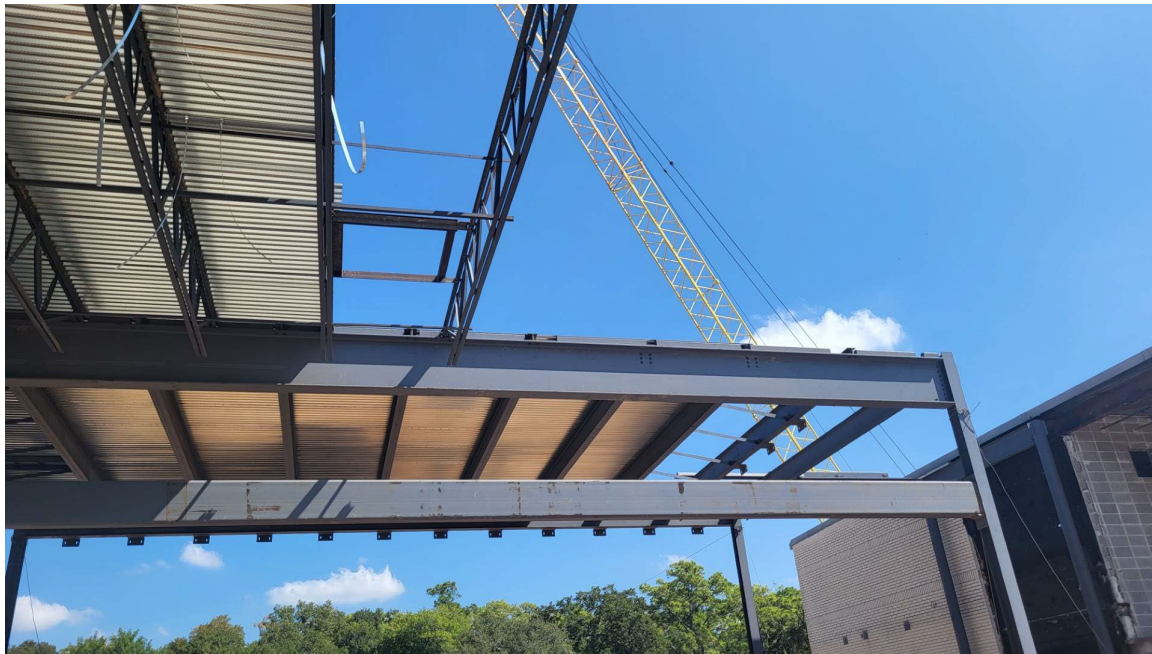
Area F Steel and Roof Deck Partial complete above Dining/Stage
