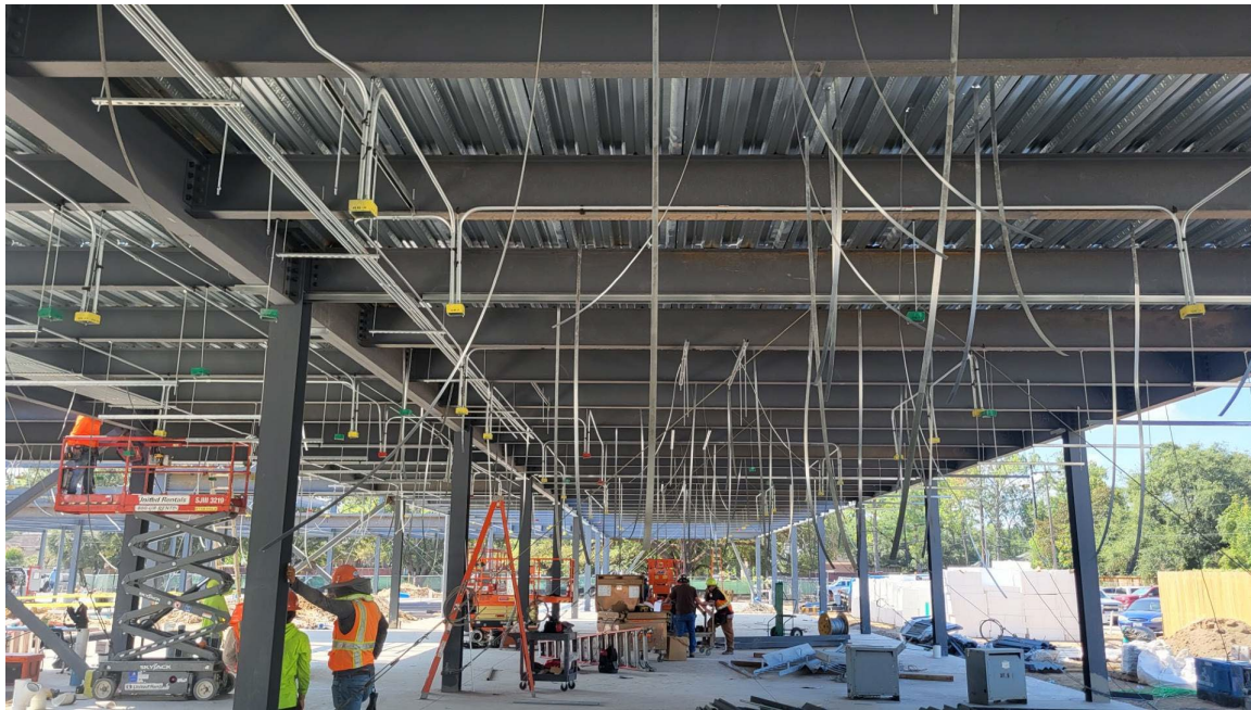
Area A with 2 nd floor deck above and duct hangers installed
