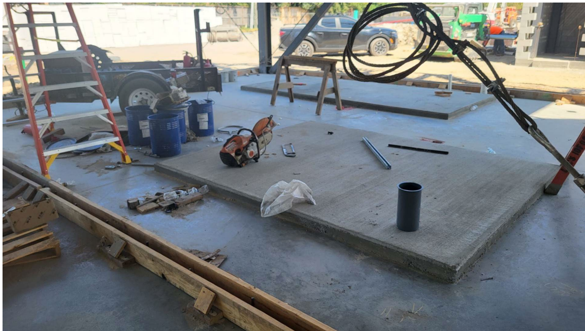
Area A Mechanical Room wall forming with equipment pads
