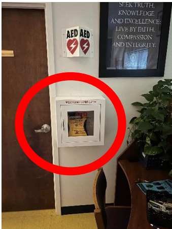
The St. Paul's School's Maintenance Building: Located behind main desk at side entrance door.
