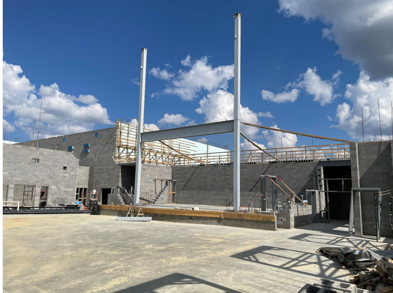
Area E - Steel Set at Stage
