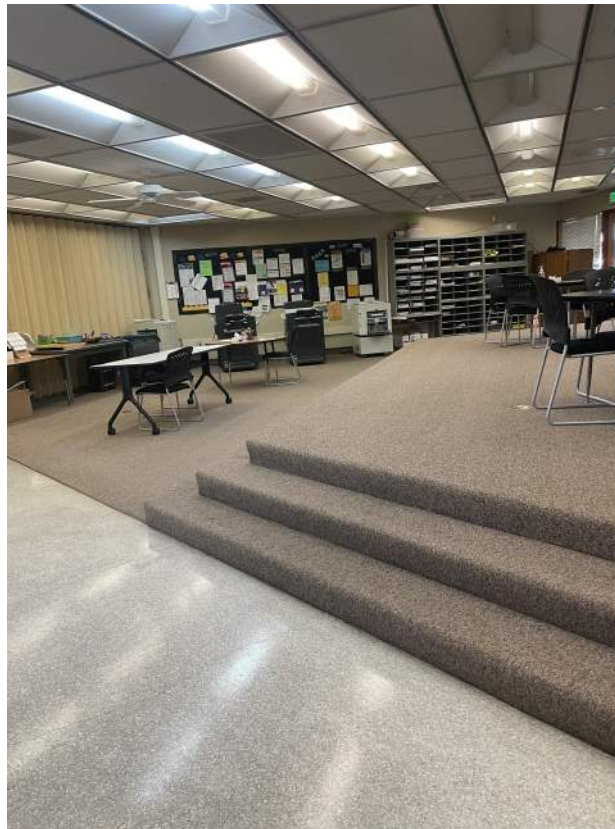
Image 2.3.6 Non-accessible MPR stage. Taken on 04/27/2022 by Belli Architectural Group.
