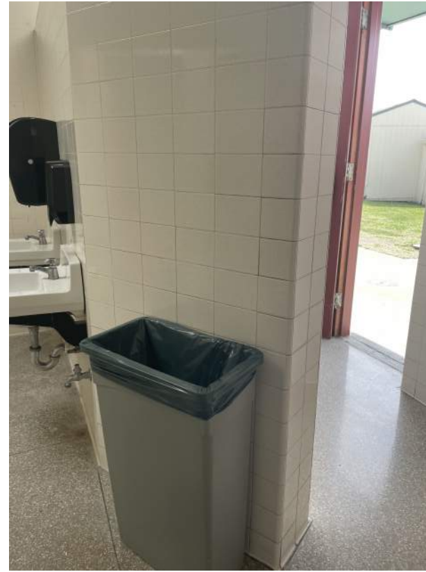
Image 2.4.1 Non-compliant clearances Taken on 04/27/2022 by Belli Architectural Group.
