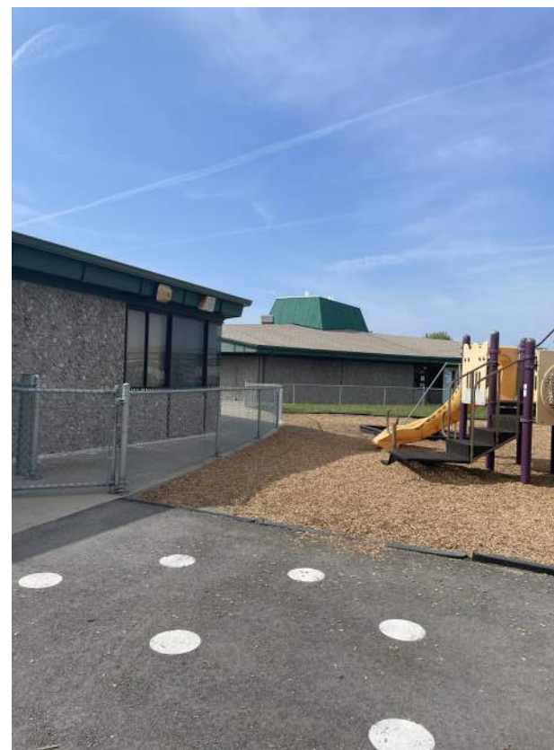
Image 2.1.3 Kindergarten playground. Taken on 04/27/2022 by Belli Architectural Group.
