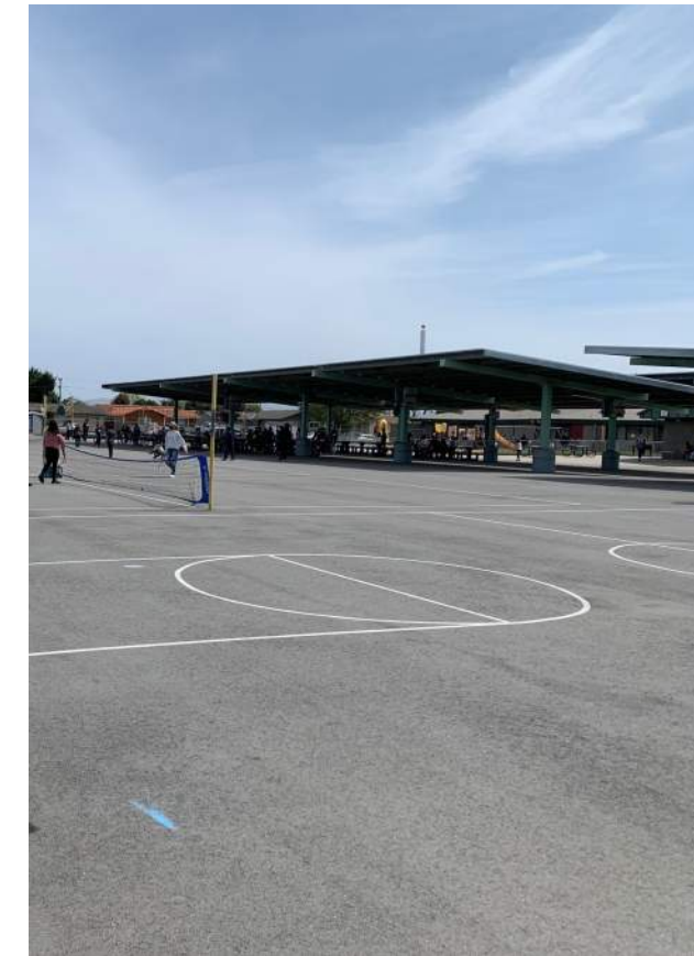
Image 2.1.4 Asphalt surfaces. Taken on 04/27/2022 by Belli Architectural Group.
