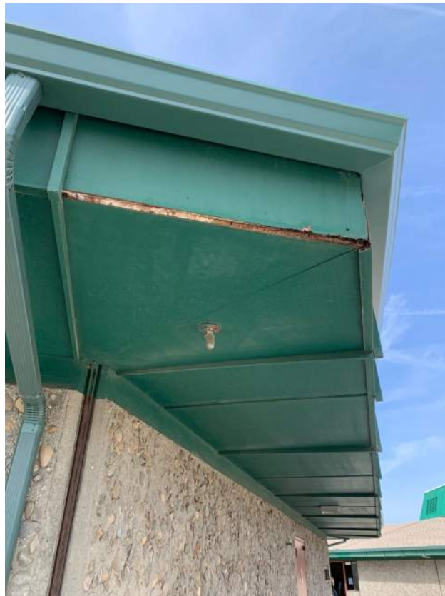
Image 2.2.1 Permanent building plywood soffits. Taken on 04/27/2022 by Belli Architectural Group.
