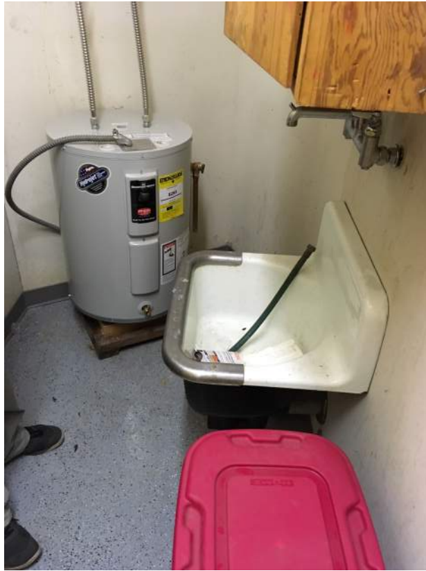
Image 2.3.11 Janitorial room. Taken on 04/27/2022 by Belli Architectural Group.
