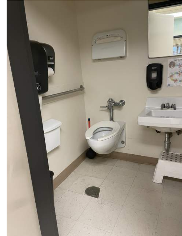
Image 2.3.9 Adult plumbing sized fixtures used by children. Taken on 04/27/2022 by Belli Architectural Group.
