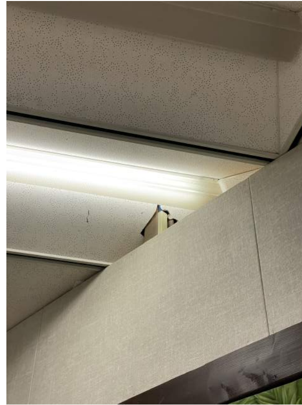
Image 2.3.7 Room partitions. Taken on 04/27/2022 by Belli Architectural Group.
