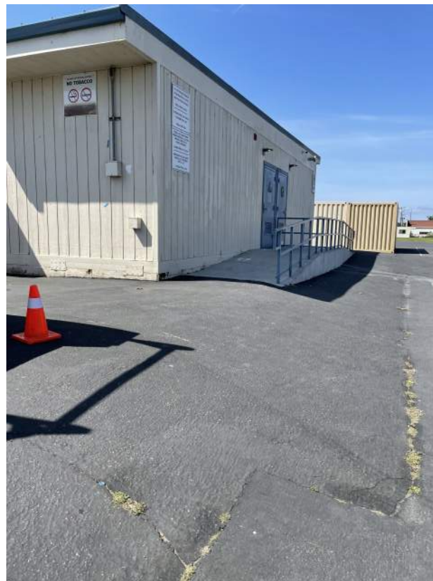
Image 2.1.2 Steep slopes on asphalt paving. Taken on 05/02/2022 by Belli Architectural Group.
