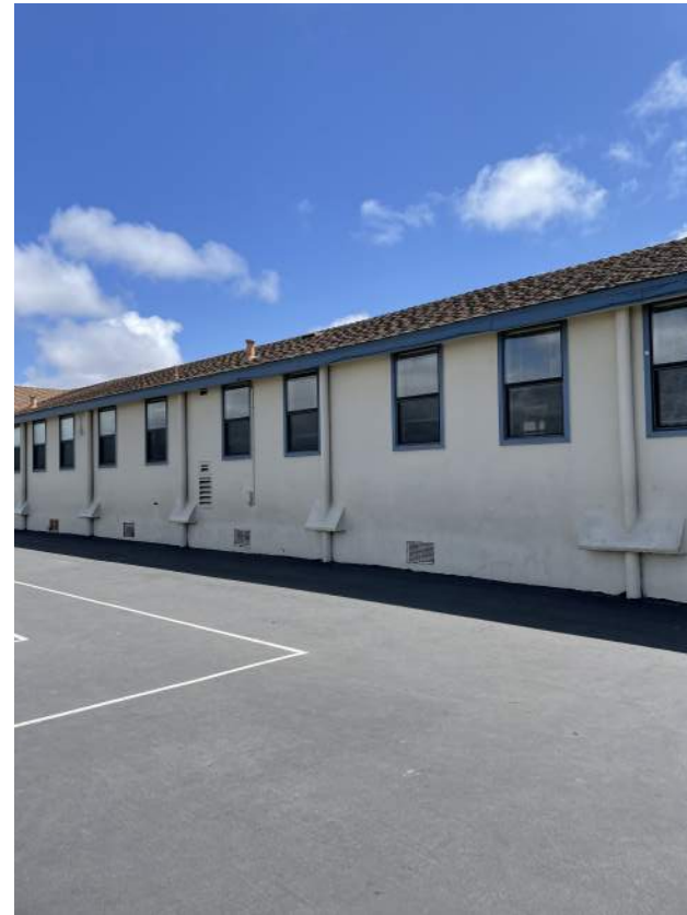
Image 2.2.6 Building B, exterior. Taken on 05/02/2022 by Belli Architectural Group.
