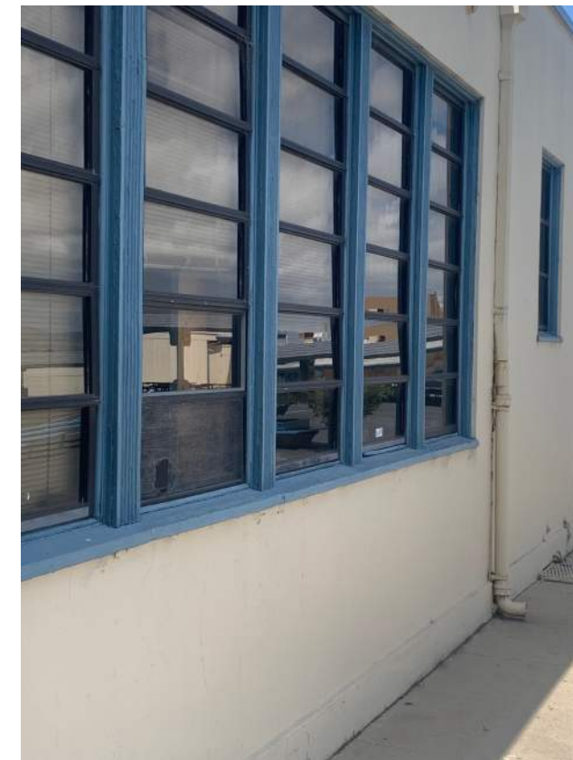
Image 2.2.2 Building A, windows. Taken on 05/02/2022 by Belli Architectural Group.
