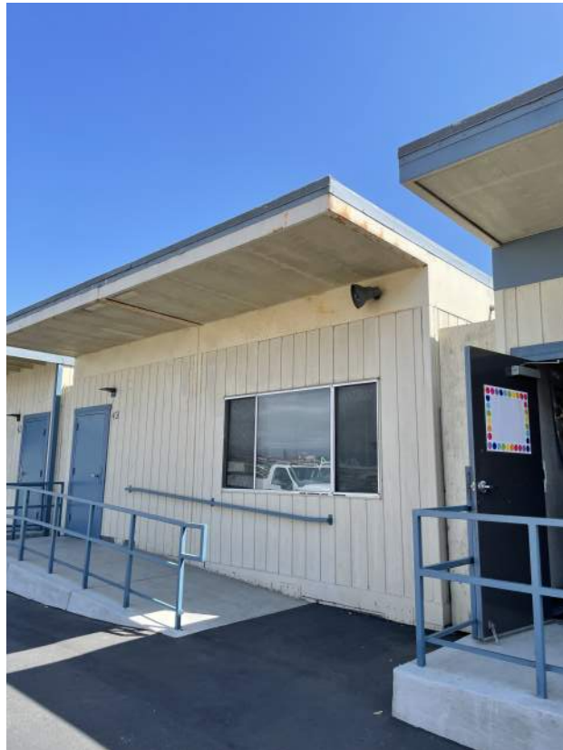
Image 2.2.15 Relocatable classroom exterior. Taken on 05/02/2022 by Belli Architectural Group.
