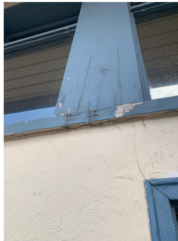
Image 2.2.13 Building D, windows. Taken on 05/02/2022 by Belli Architectural Group.
