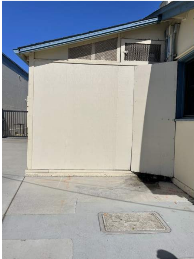
Image 2.3.19 Kitchen addition. Taken on 06/29/2022 by Belli Architectural Group.
