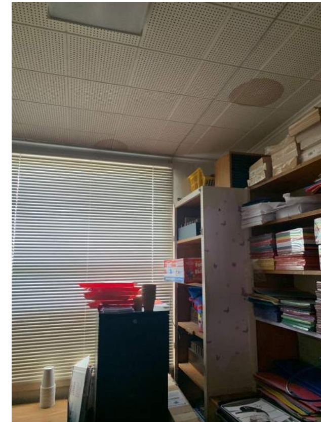
Image 2.3.6 Building C, ceiling panels. Taken on 05/02/2022 by Belli Architectural Group.
