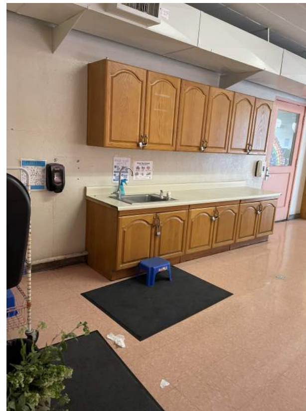
Image 2.3.10 Building C, sinks. Taken on 05/02/2022 by Belli Architectural Group.
