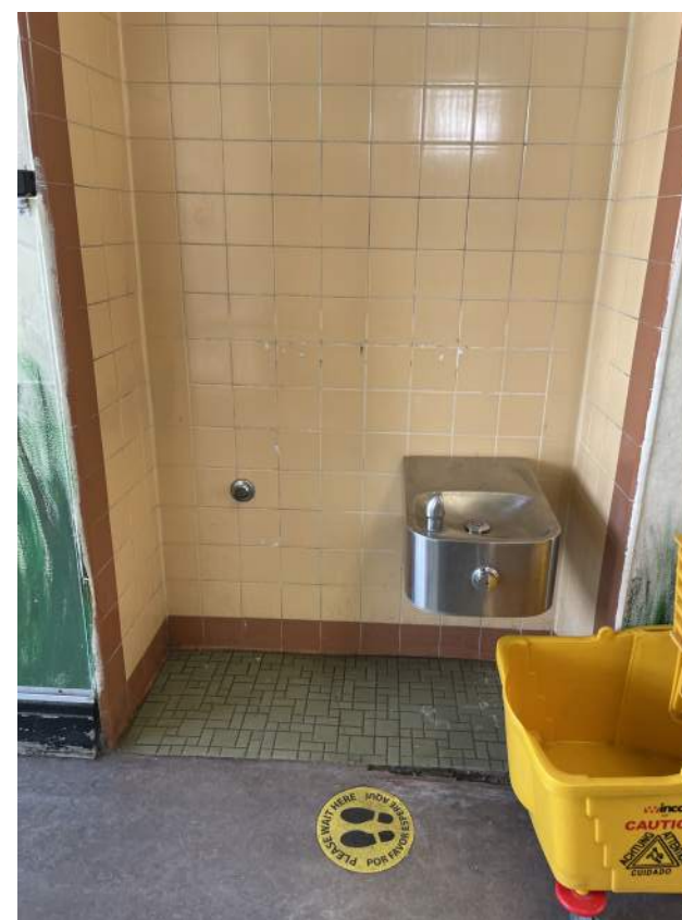
Image 2.3.16 Building E, water fountain. Taken on 05/02/2022 by Belli Architectural Group.
