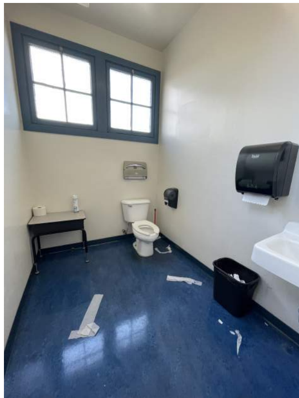
Image 2.3.3 Building A, single occupancy restrooms. Taken on 05/02/2022 by Belli Architectural Group.
