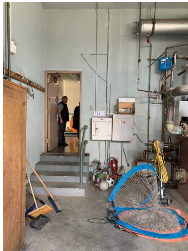
Image 2.3.14 Building E, machinery. Taken on 05/02/2022 by Belli Architectural Group.
