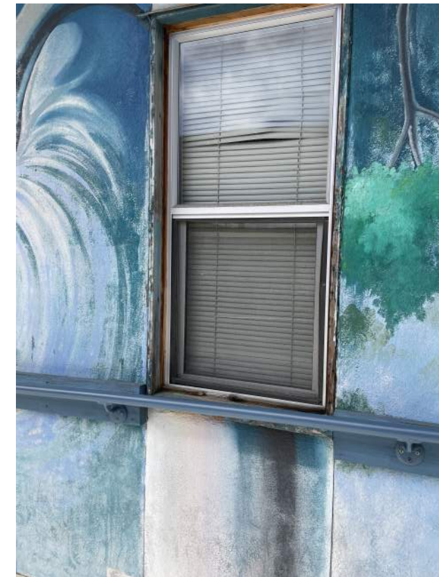
Image 2.2.14 Building F, windows. Taken on 05/02/2022 by Belli Architectural Group.
