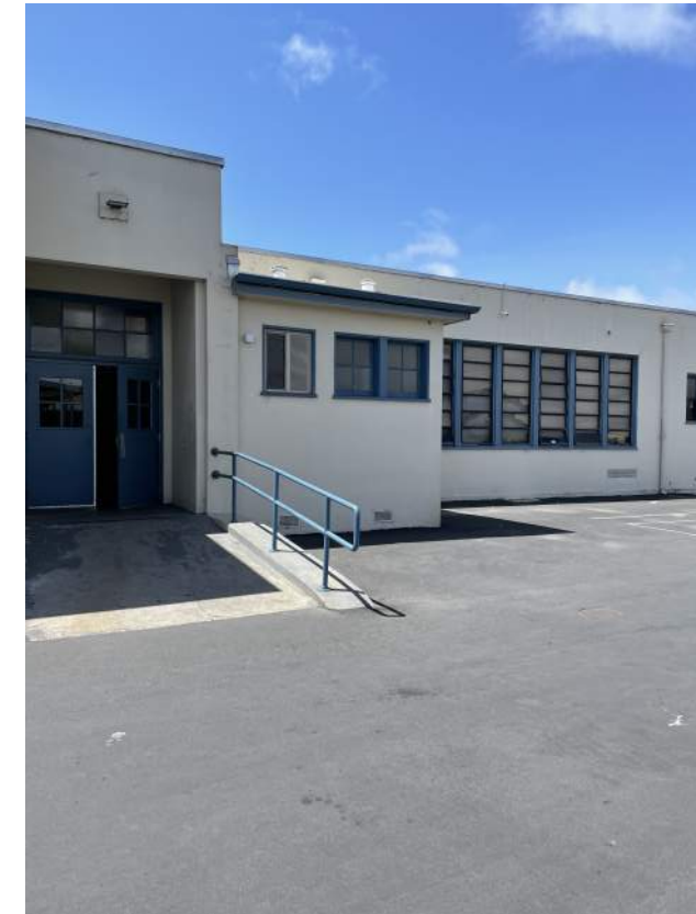
Image 2.2.1 Building A, exterior. Taken on 05/02/2022 by Belli Architectural Group.
