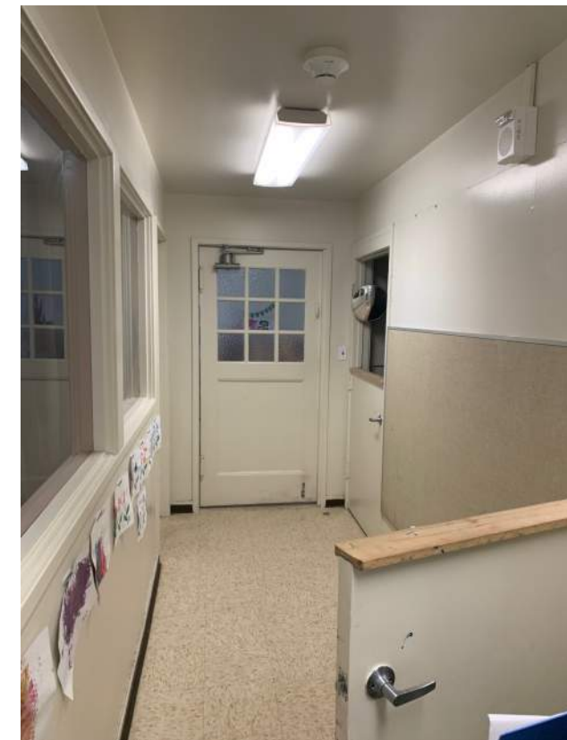
Image 2.3.7 Building C, wall finishes. Taken on 05/02/2022 by Belli Architectural Group.
