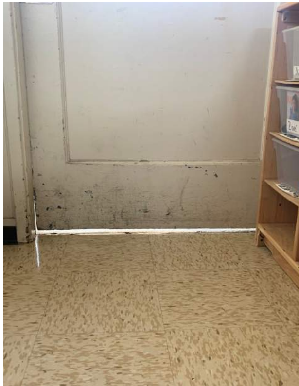
Image 2.3.8 Building C, doors. Taken on 05/02/2022 by Belli Architectural Group.
