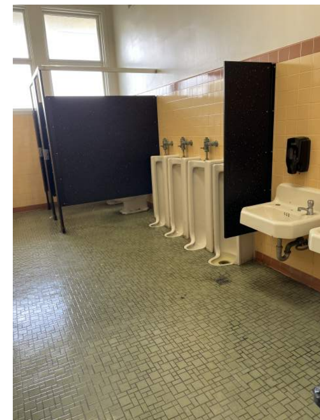
Image 2.3.12 Building E, restrooms. Taken on 05/02/2022 by Belli Architectural Group.
