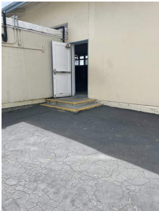
Image 2.2.11 Building D, non-accessible entry. Taken on 05/02/2022 by Belli Architectural Group.
