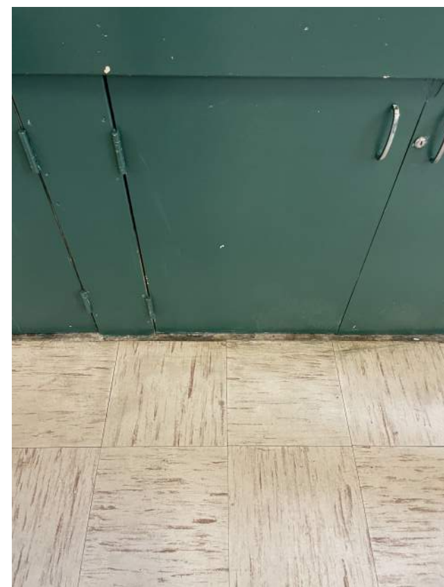
Image 2.3.8 Relocatable building floor. Taken on 04/27/2022 by Belli Architectural Group.
