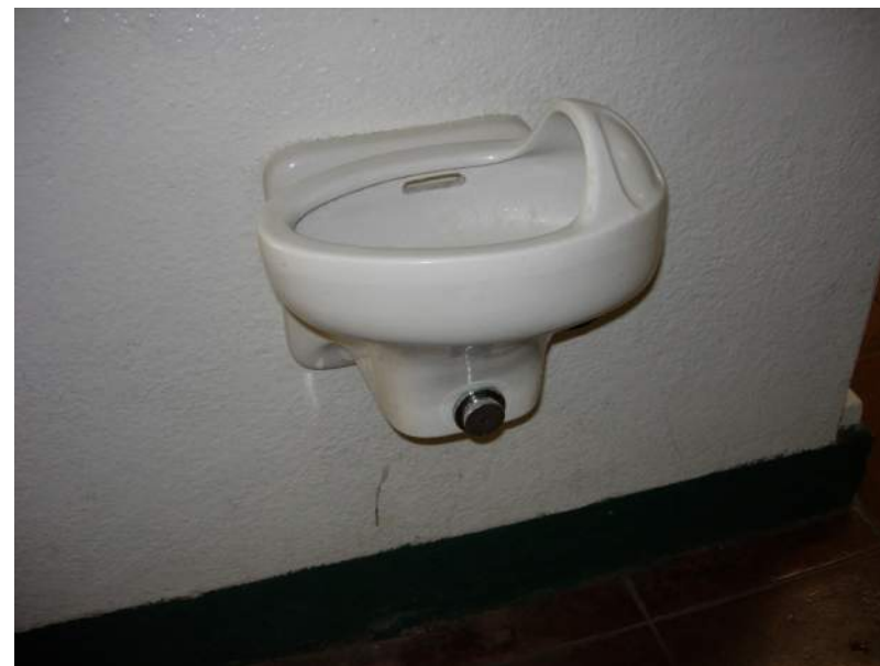
A typical wall mounted drinking fountain that does not meet ADA and should be replaced.
