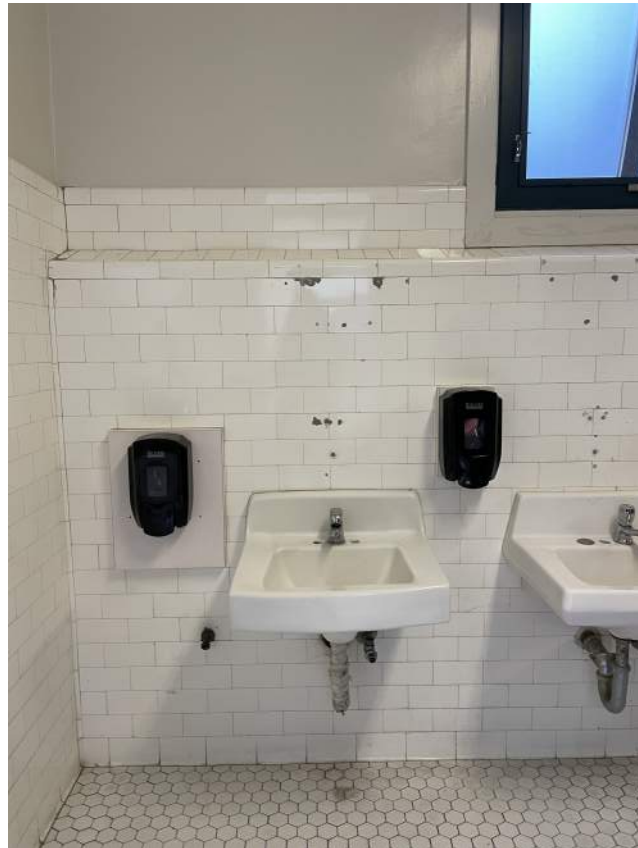
Image 2.3.5 Existing restrooms. Taken on 04/27/2022 by Belli Architectural Group.
