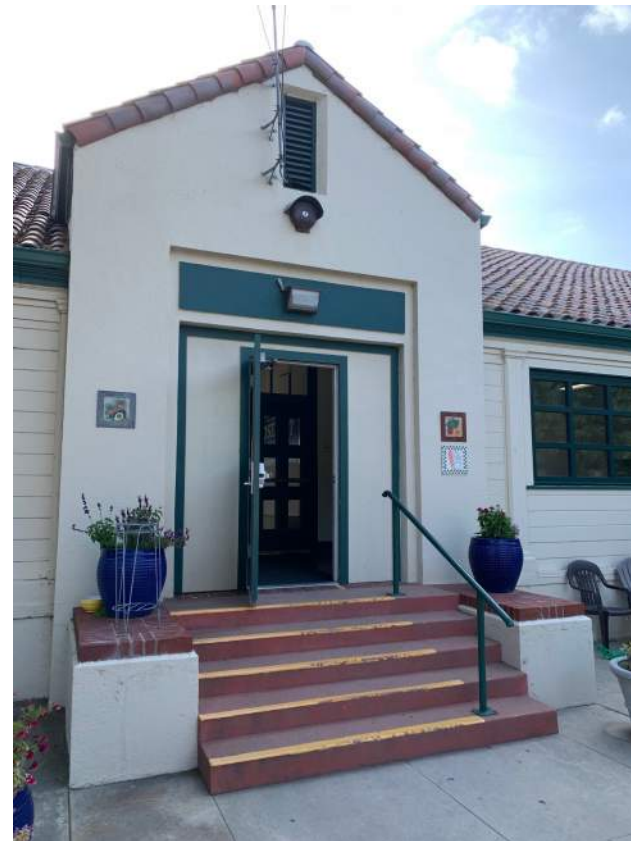
Image 2.1.2 No access ramp at courtyard. Taken on 04/27/2022 by Belli Architectural Group.
