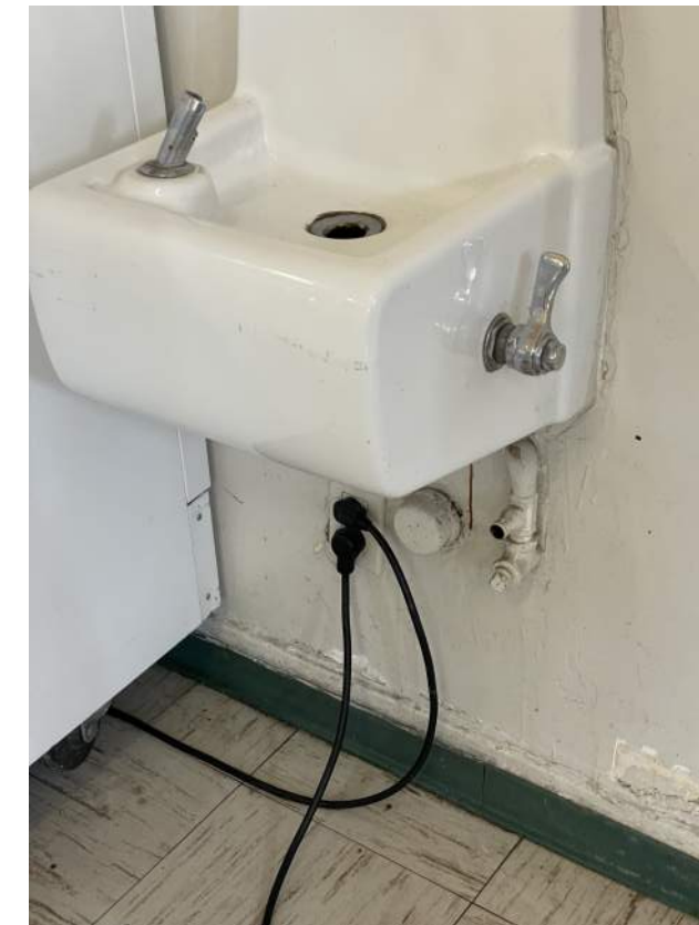
Image 2.3.3 Outlets under drinking fountain. Taken on 04/27/2022 by Belli Architectural Group.
