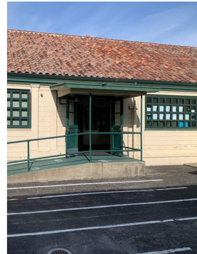
Image 2.2.3 Original building roof. Taken on 04/27/2022 by Belli Architectural Group.
