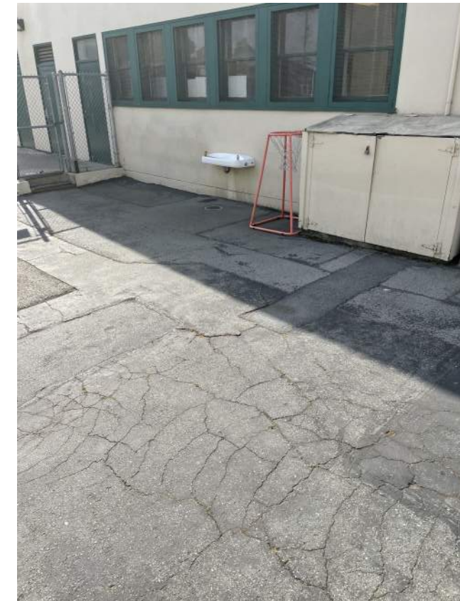
Image 2.2.2 MPR exterior. Taken on 04/27/2022 by Belli Architectural Group.
