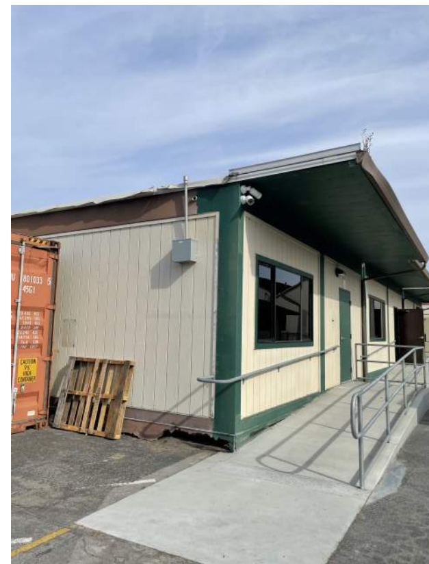
Image 2.2.6 Relocatable classroom. Taken on 04/27/2022 by Belli Architectural Group.
