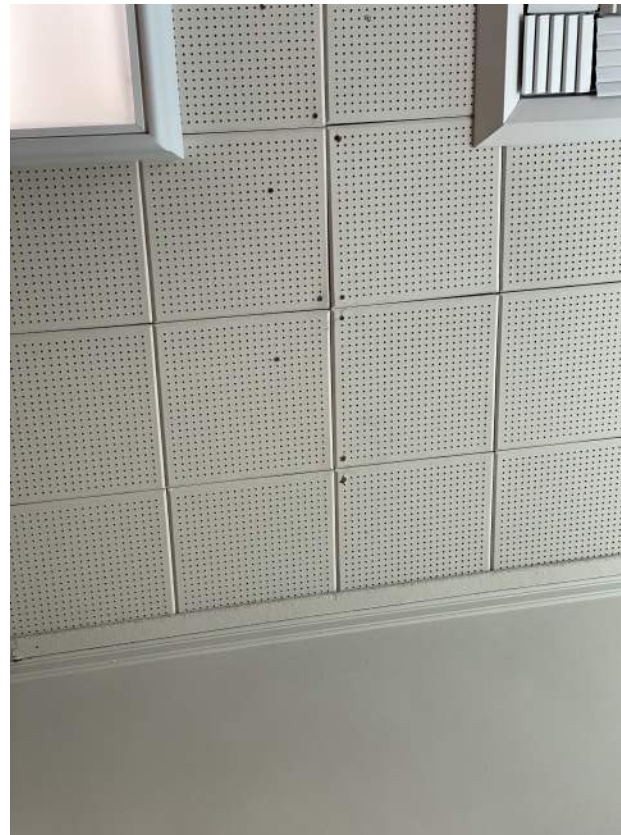
Image 2.3.1 Acoustic ceiling panels. Taken on 04/27/2022 by Belli Architectural Group.
