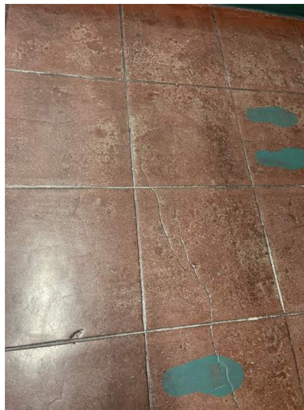
Image 2.3.2 Hallway flooring. Taken on 04/27/2022 by Belli Architectural Group.
