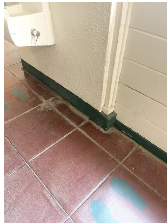
Image 2.4.2 Drinking fountain. Taken on 04/27/2022 by Belli Architectural Group.
