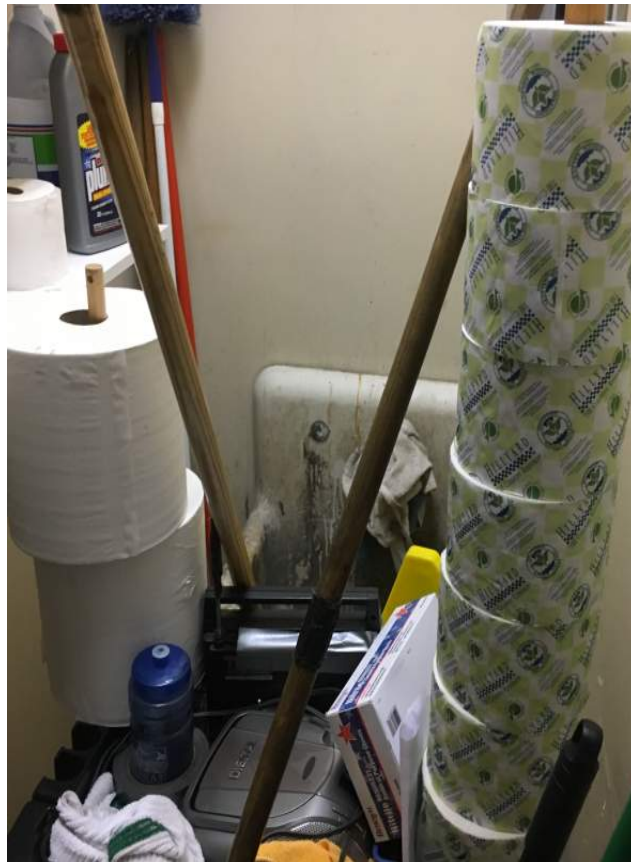
Image 2.3.12 Janitorial room. Taken on 04/27/2022 by Belli Architectural Group.
