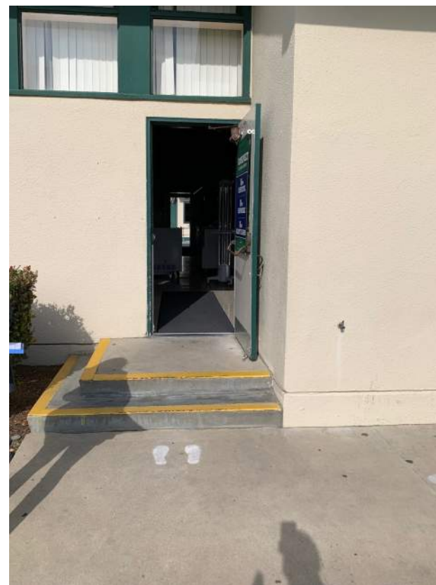
Image 2.1.3 Non-accessible entrance and unlocked door from MPR to street. Taken on 04/27/2022 by Belli Architectural Group.
