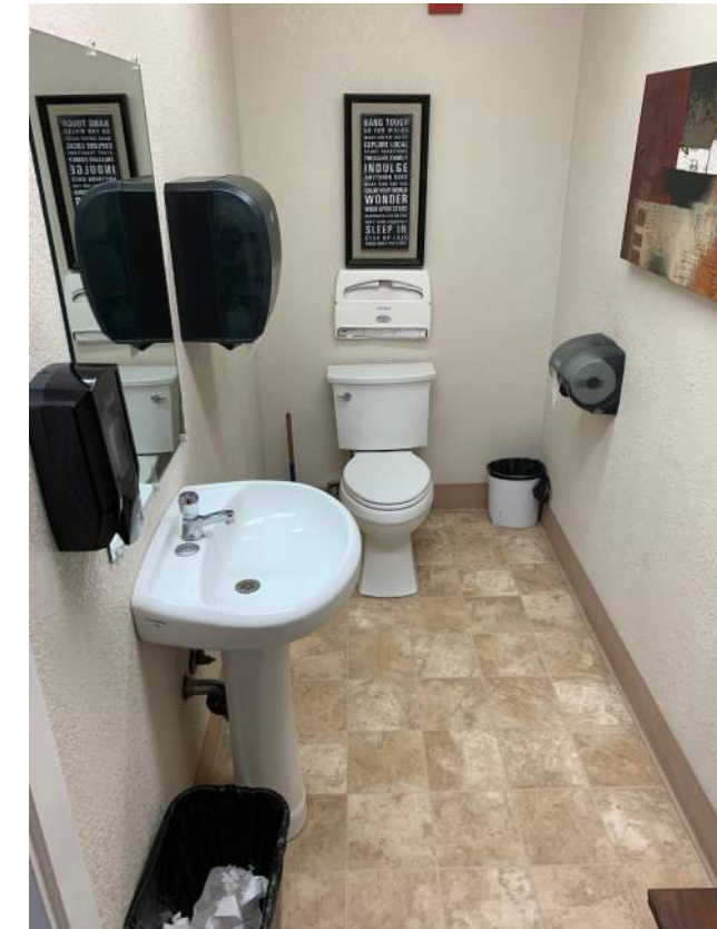
Image 2.4.4 Small, non-accessible single occupancy restroom. Taken on 04/27/2022 by Belli Architectural Group.
