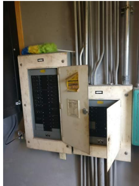
OLD ORIGINAL PANELS.
