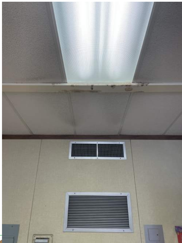
Image 2.3.6 Relocatable building ceiling and wall. Taken on 04/27/2022 by Belli Architectural Group.
