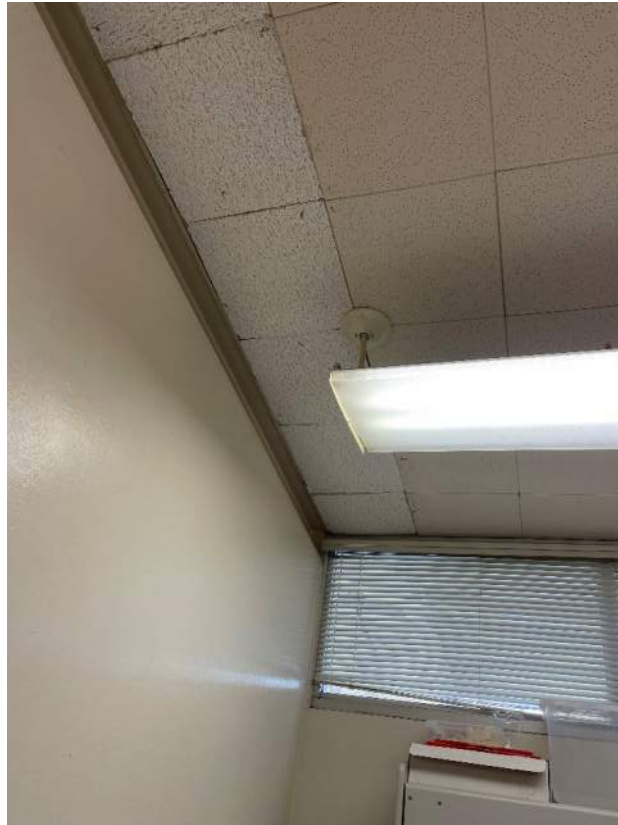
Image 2.3.3 Ceiling panels. Taken on 05/02/2022 by Belli Architectural Group.
