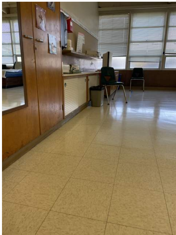
Image 2.3.4 VCT flooring and existing casework. Taken on 05/02/2022 by Belli Architectural Group.
