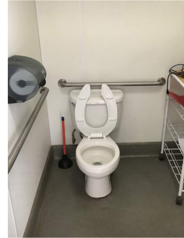
Image 2.3.7 Preschool restrooms. Taken on 05/02/2022 by Belli Architectural Group.
