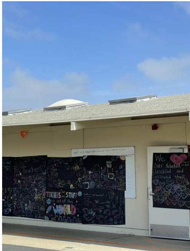
Image 2.2.1 Permanent building roof. Taken on 05/02/2022 by Belli Architectural Group.
