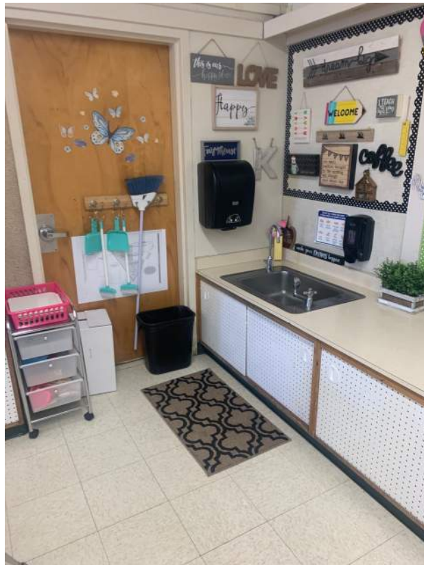
Image 2.4.1 Non-accessible classroom sink. Taken on 05/02/2022 by Belli Architectural Group.
