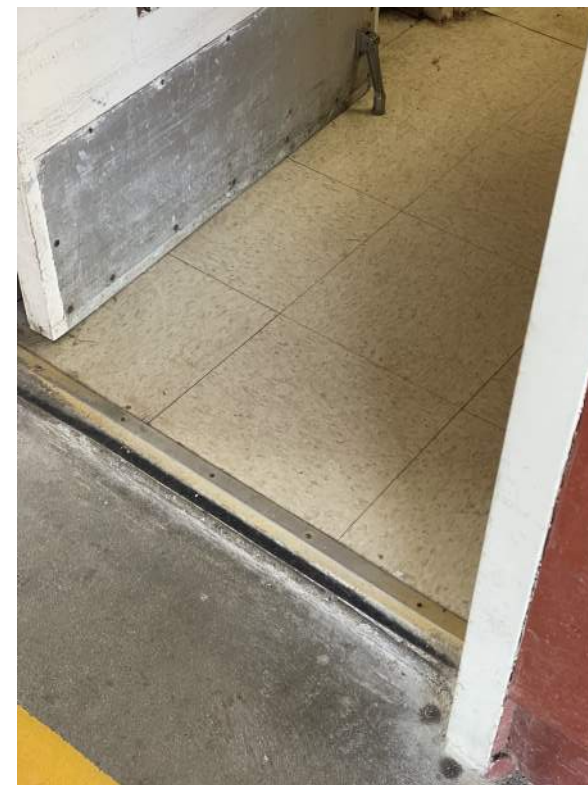
Image 2.4.3 Non-compliant threshold. Taken on 04/27/2022 by Belli Architectural Group.
