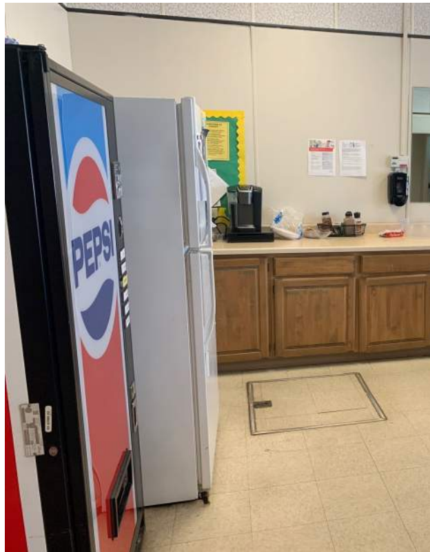
Image 2.3.3 Patched sheet vinyl flooring at under-floor access panel. Taken on 04/27/2022 by Belli Architectural Group.
