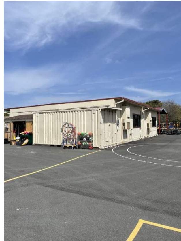
Image 2.2.7 Storage container next to classroom. Taken on 04/27/2022 by Belli Architectural Group.
