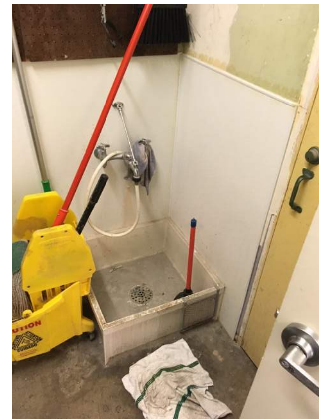
Image 2.3.8 Janitorial room. Taken on 04/27/2022 by Belli Architectural Group.
