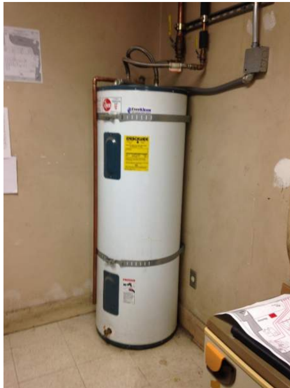
Restroom Building near Classroom 1:
