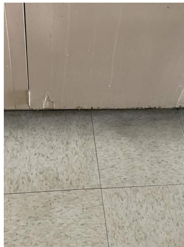
Image 2.3.6 Classroom casework. Taken on 04/27/2022 by Belli Architectural Group.
