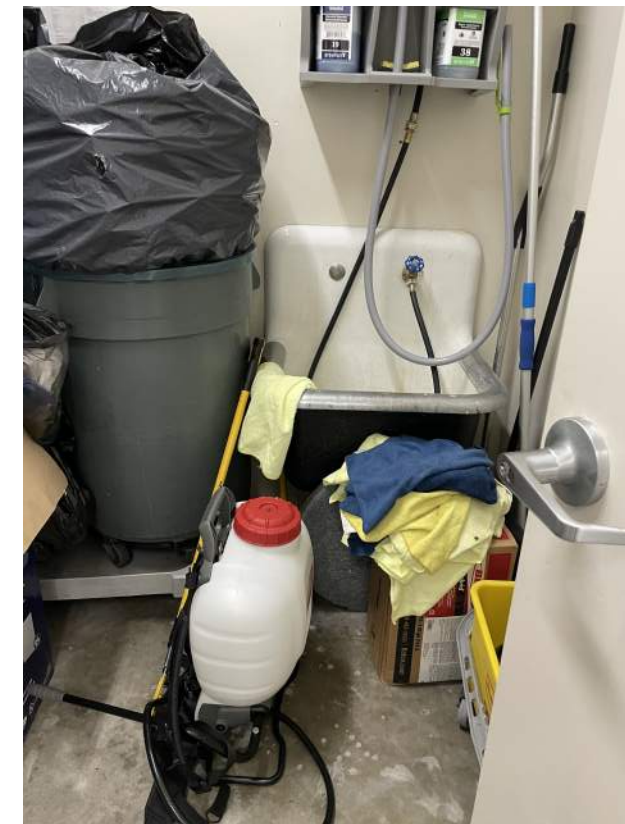
Image 2.3.15 Janitorial Room. Taken on 06/29/2022 by Belli Architectural Group.
