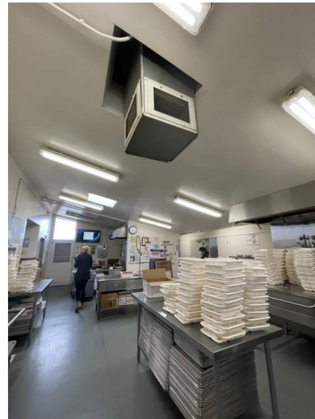
Image 2.3.13 Kinchen equipment. Taken on 06/29/2022 by Belli Architectural Group.
