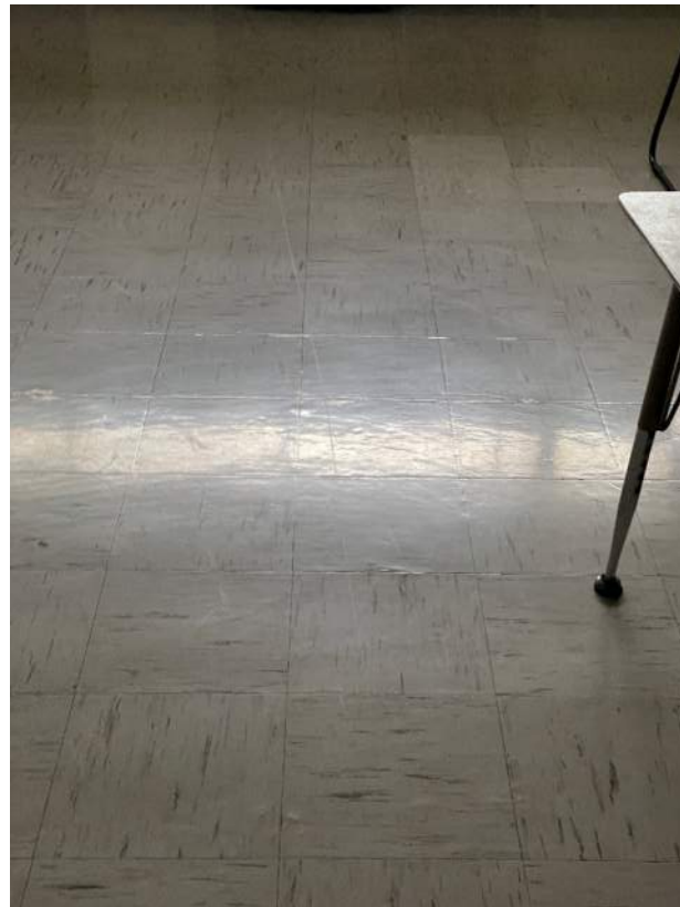
Image 2.3.5 Old VCT floor. Taken on 04/27/2022 by Belli Architectural Group.
