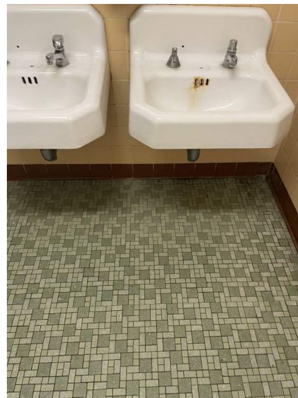
Image 2.3.8 Rust at plumbing fixtures. Taken on 04/27/2022 by Belli Architectural Group.
