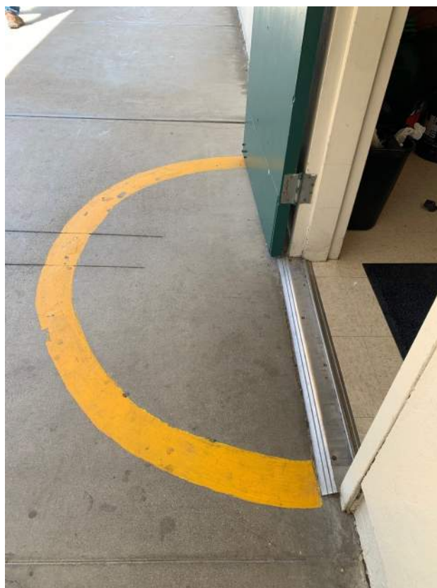
Image 2.2.3 Threshold. Taken on 05/03/2022 by Belli Architectural Group.
