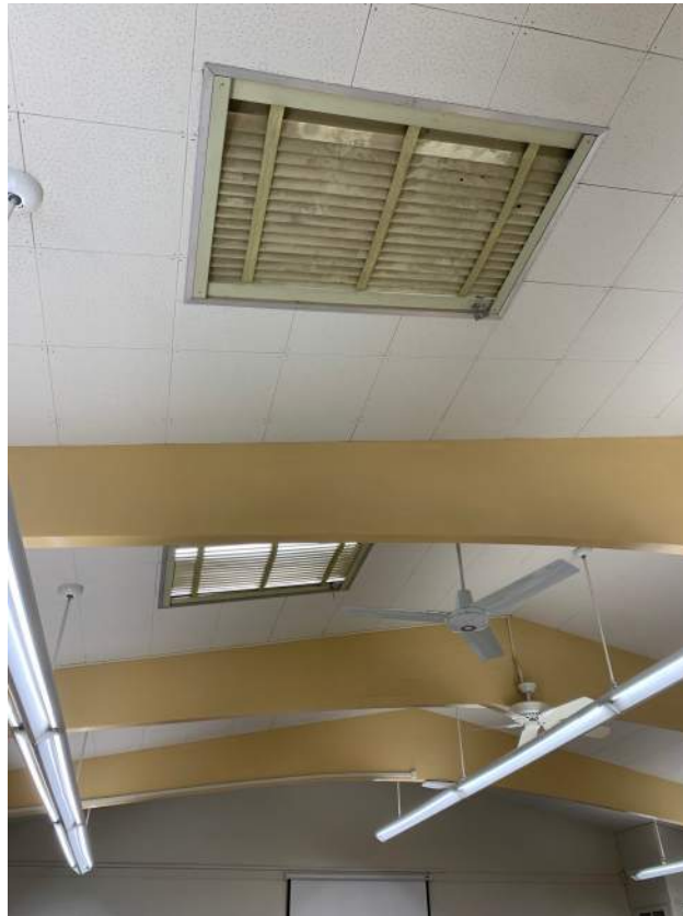
Image 2.3.1 Dirty louvers at aged skylights. Taken on 05/03/2022 by Belli Architectural Group.
