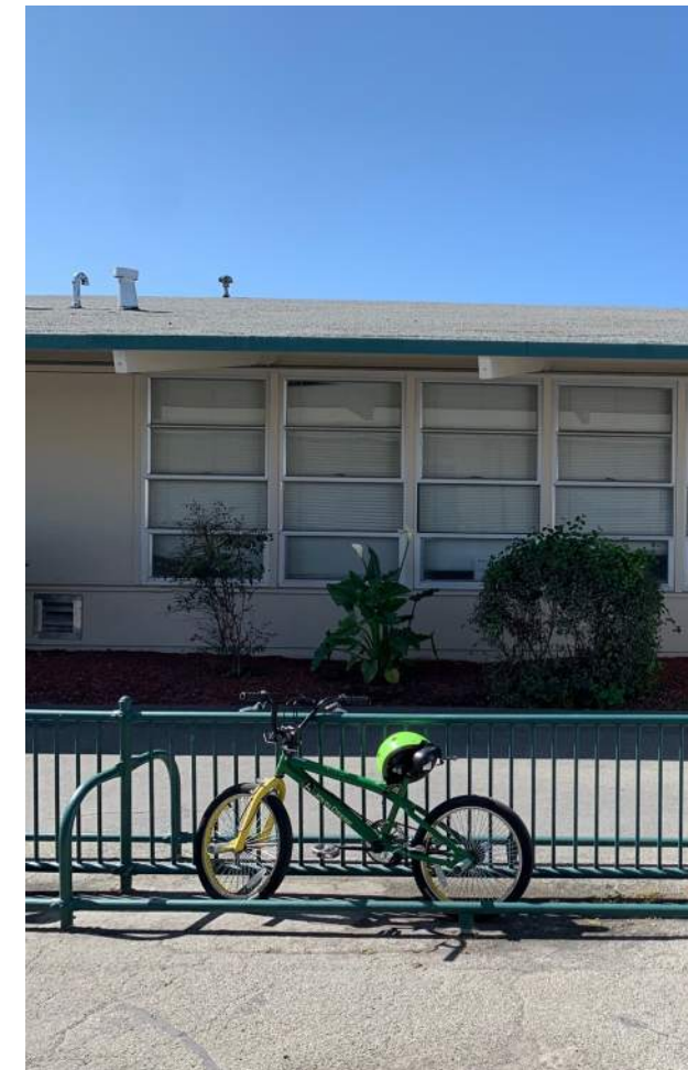
Image 2.2.1 Permanent classroom roof. Taken on 05/03/2022 by Belli Architectural Group.
