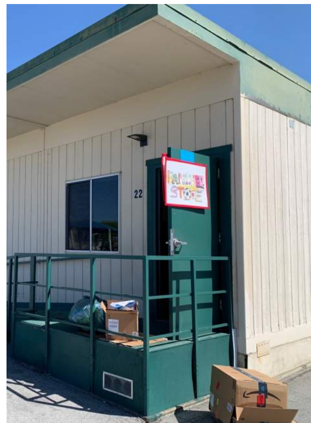
Image 2.2.5 Relocatable classroom exterior. Taken on 05/03/2022 by Belli Architectural Group.
