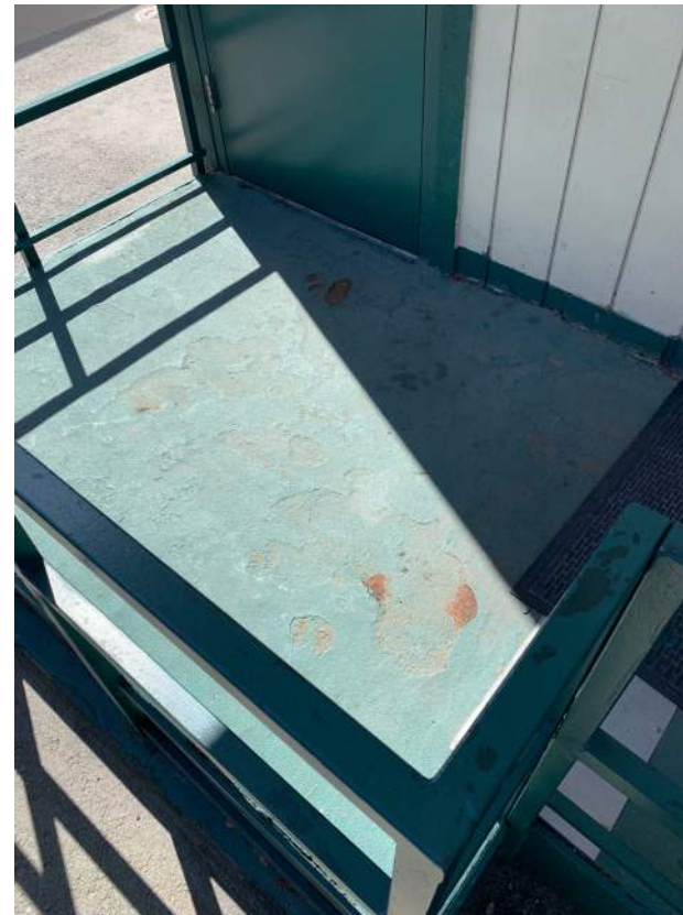
Image 2.2.4 Relocatable classroom access ramp. Taken on 05/03/2022 by Belli Architectural Group.
