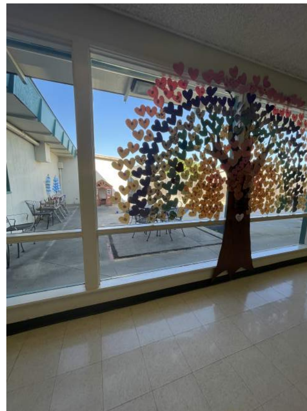
Image 2.2.3 Original windows at admin. office. Taken on 05/03/2022 by Belli Architectural Group.
