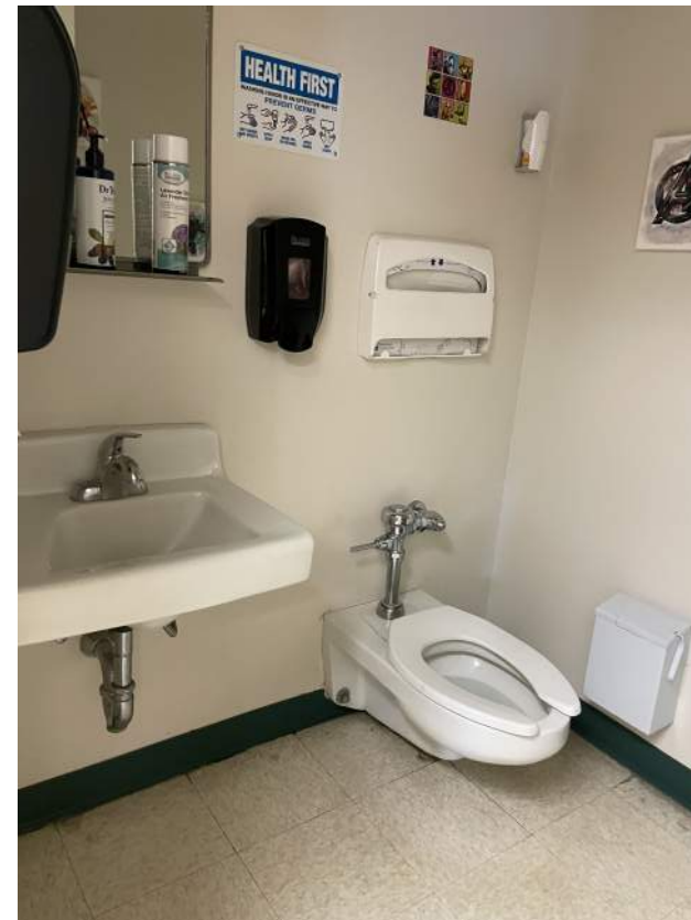
Image 2.4.2 Non-ADA compliant restroom and accessories. Taken on 05/03/2022 by Belli Architectural Group.
