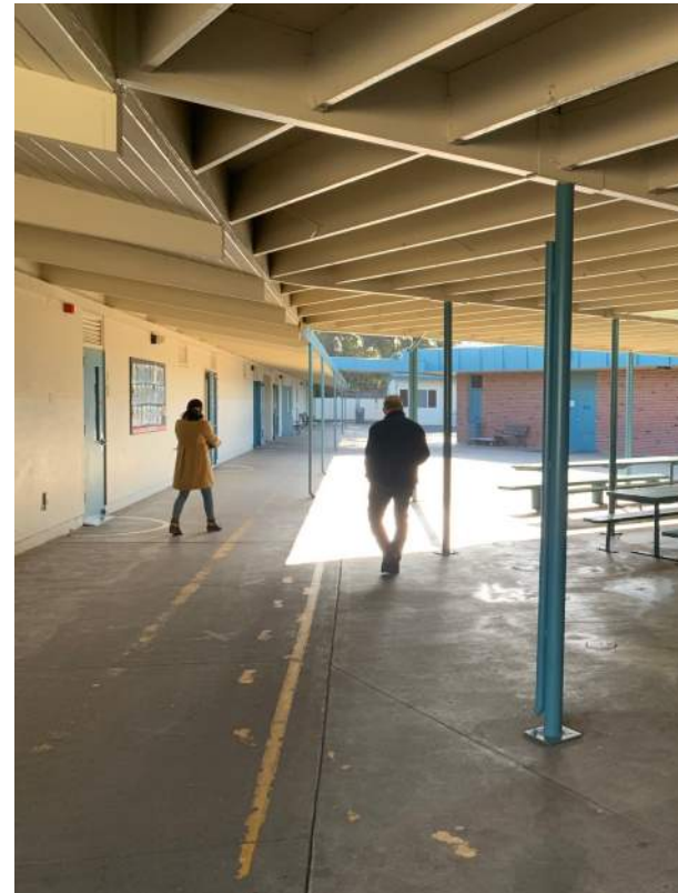
Image 2.1.2 Site paint striping. Taken on 05/03/2022 by Belli Architectural Group.
