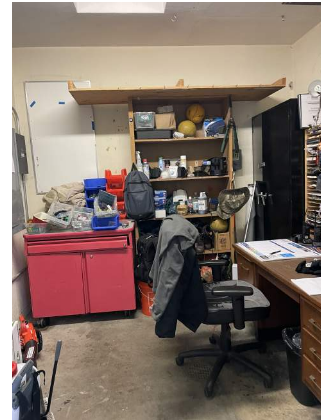
Image 2.3.10 Janitorial Room. Taken on 05/03/2022 by Belli Architectural Group.
