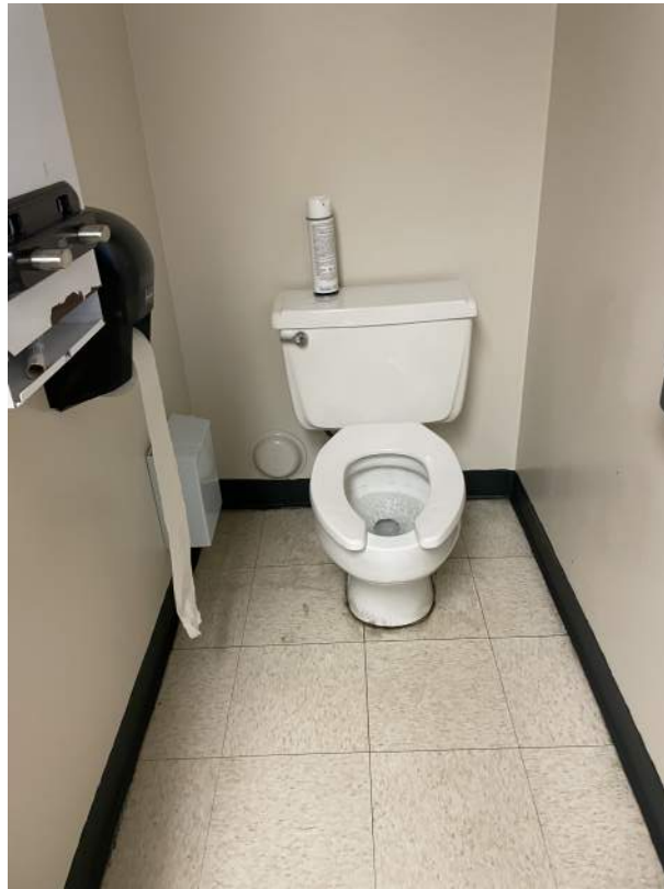
Image 2.3.6 Single occupancy non-accessible restroom. Taken on 05/03/2022 by Belli Architectural Group.
