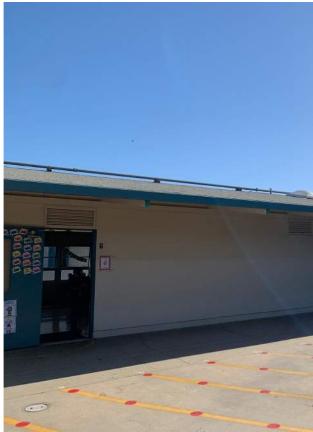
Image 2.2.1 Permanent building gravel roof. Taken on 05/03/2022 by Belli Architectural Group.
