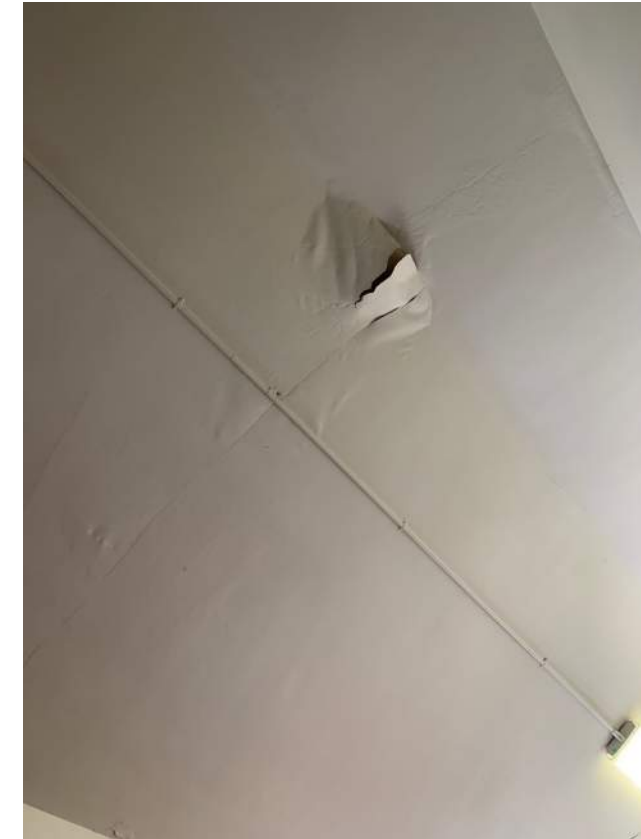
Image 2.3.9 Relocatable classroom ceiling. Taken on 05/03/2022 by Belli Architectural Group.
