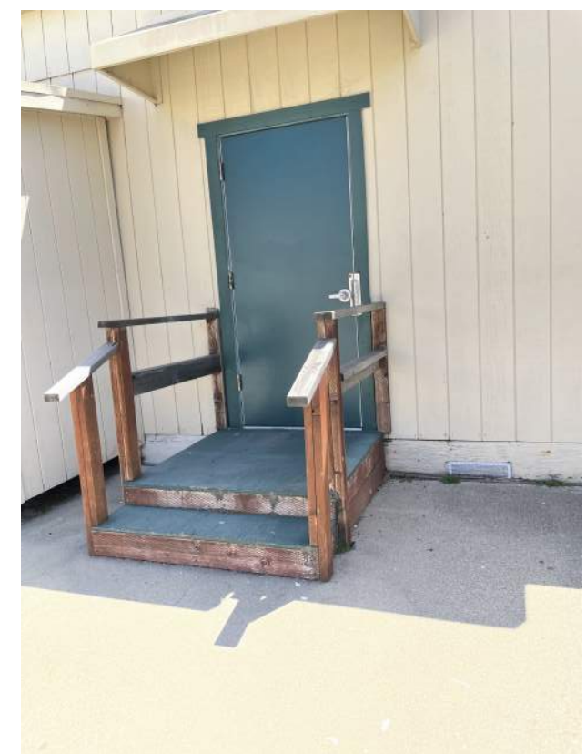
Image 2.2.8 Non-accessible stairs to relocatable building. Taken on 05/03/2022 by Belli Architectural Group.
