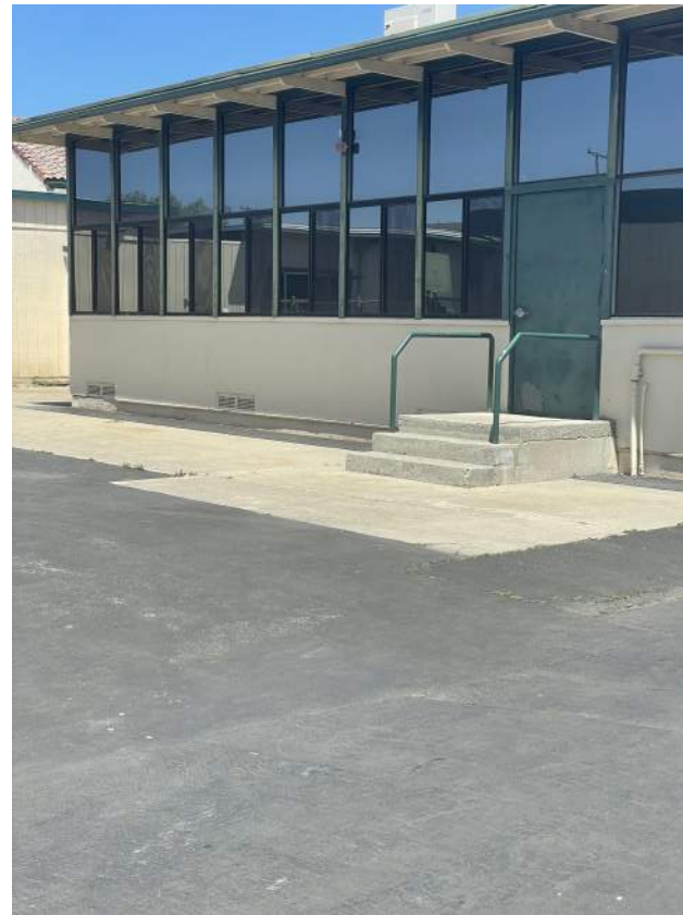
Image 2.1.2 Non-accessible relocatable building entrance. Taken on 05/03/2022 by Belli Architectural Group.
