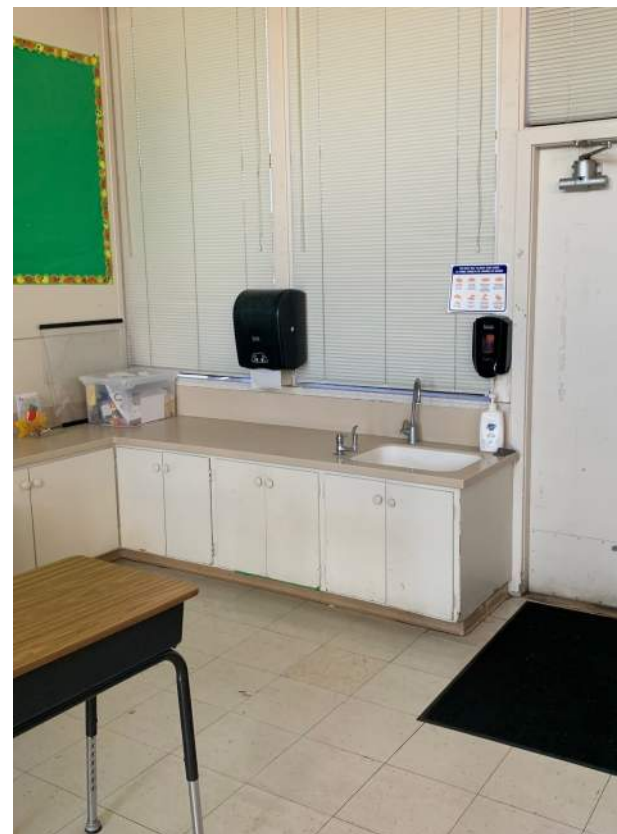
Image 2.3.8 VCT flooring. Taken on 05/03/2022 by Belli Architectural Group.
