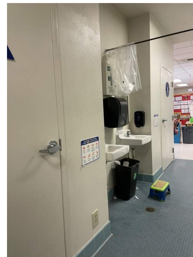
Image 2.3.5 Kindergarten sinks. Taken on 04/26/2022 by Belli Architectural Group.
