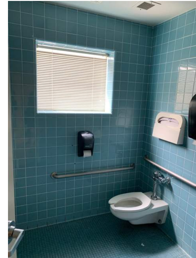
Image 2.4.2 Grab bars at different heights. Taken on 04/26/2022 by Belli Architectural Group.
