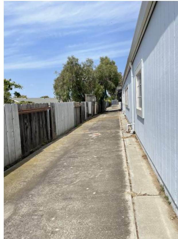
Image 2.1.2 Existing alley behind classrooms. Taken on 04/26/2022 by Belli Architectural Group.
