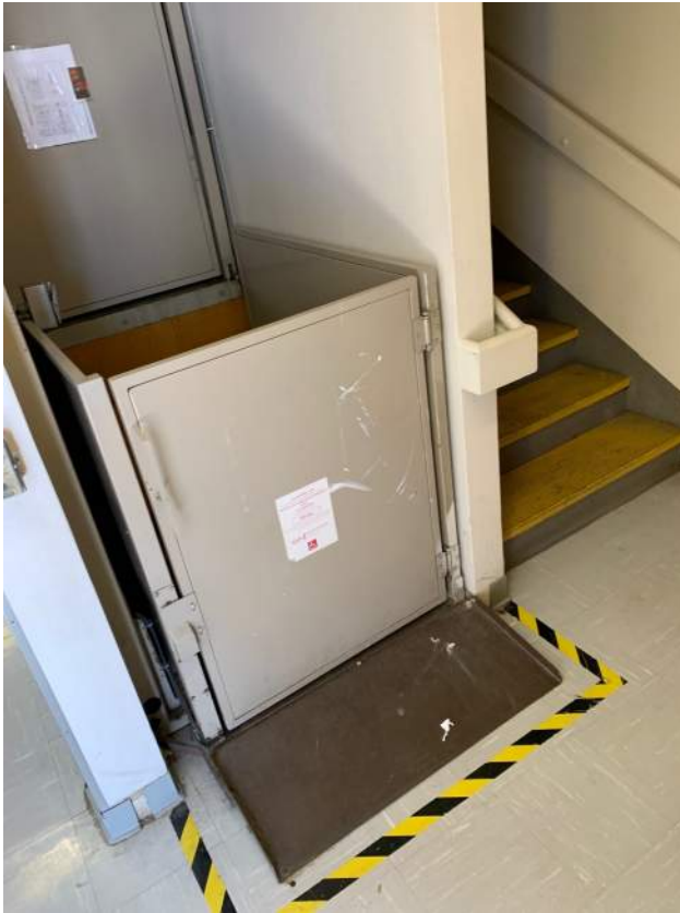
Image 2.4.4 Accessible chair lift to stage. Taken on 04/26/2022 by Belli Architectural Group.
