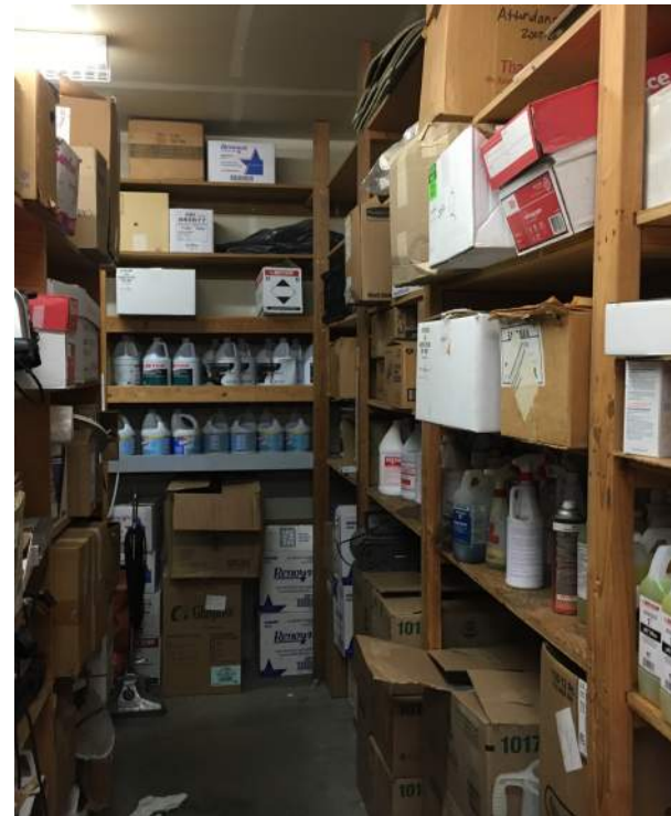
Image 2.3.16 Janitorial room. Taken on 04/26/2022 by Belli Architectural Group.
