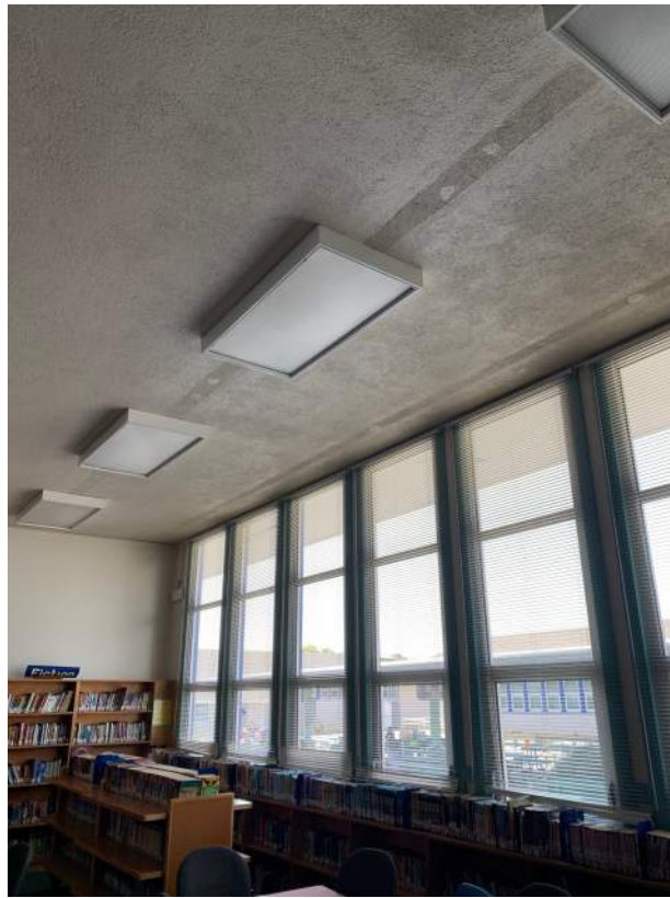
Image 2.3.3 Classroom ceiling. Taken on 04/26/2022 by Belli Architectural Group.
