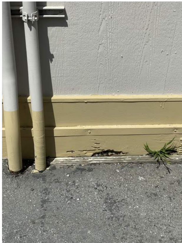
Image 2.2.1 Relocatable building wall. Taken on 04/26/2022 by Belli Architectural Group.
