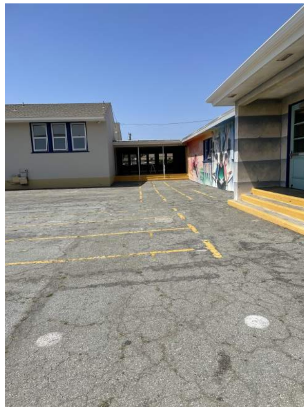
Image 2.1.1 Asphalt and striping existing conditions. Taken on 04/26/2022 by Belli Architectural Group.
