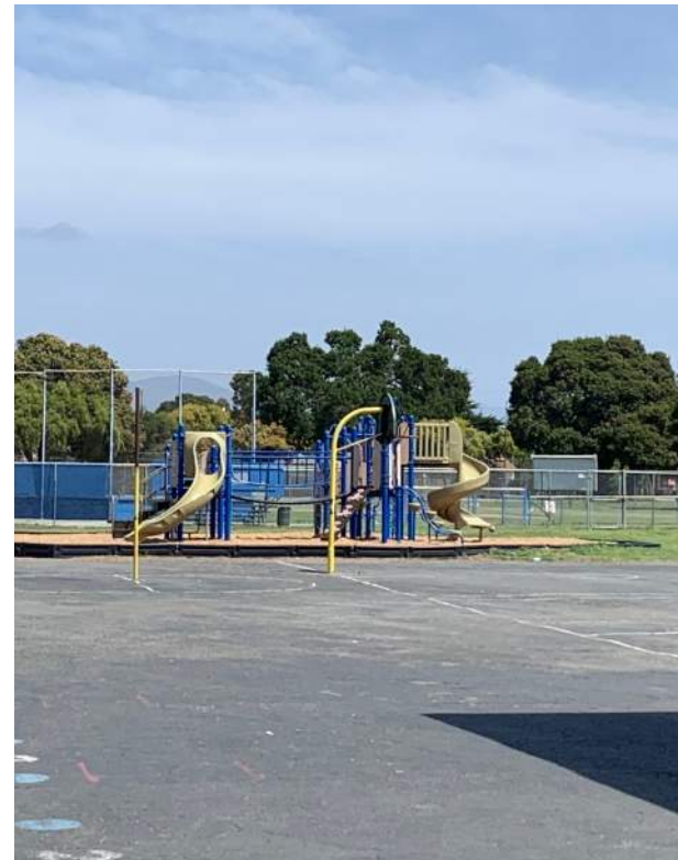
Image 2.1.2 Asphalt and striping existing conditions. Taken on 04/26/2022 by Belli Architectural Group.
