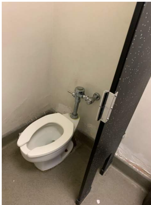
Image 2.2.4 Existing, non-accessible restroom at MPR. Taken on 04/26/2022 by Belli Architectural Group.
