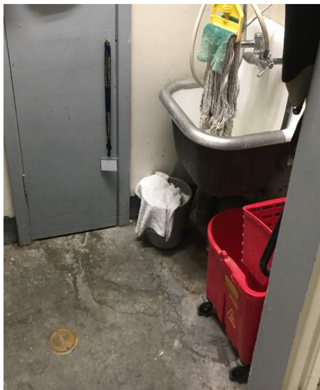
Image 2.3.12 Janitorial room. Taken on 05/02/2022 by Belli Architectural Group.
