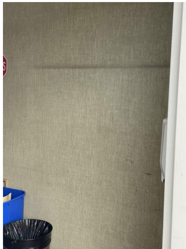
Image 2.3.2 Worn and dirty wall paper at library. Taken on 05/02/2022 by Belli Architectural Group.
