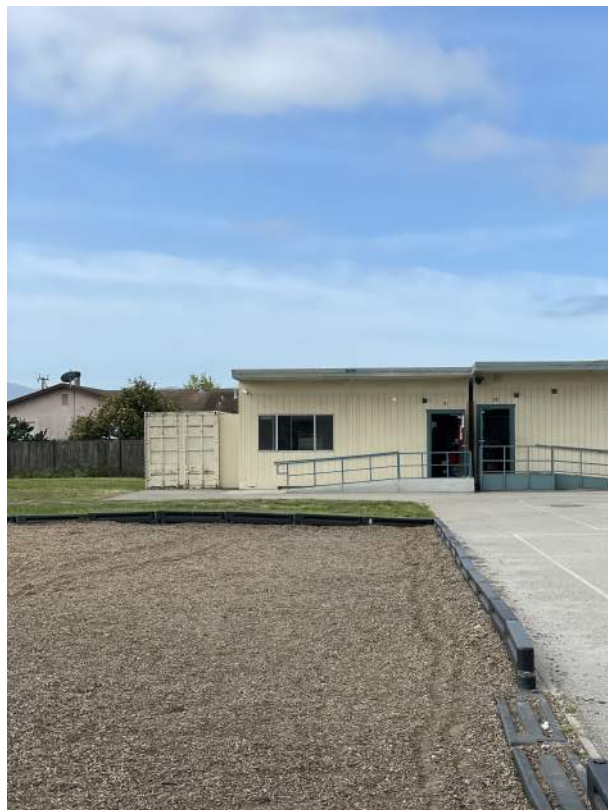
Image 2.1.1 Storage container next to classroom. Taken on 05/02/2022 by Belli Architectural Group.
