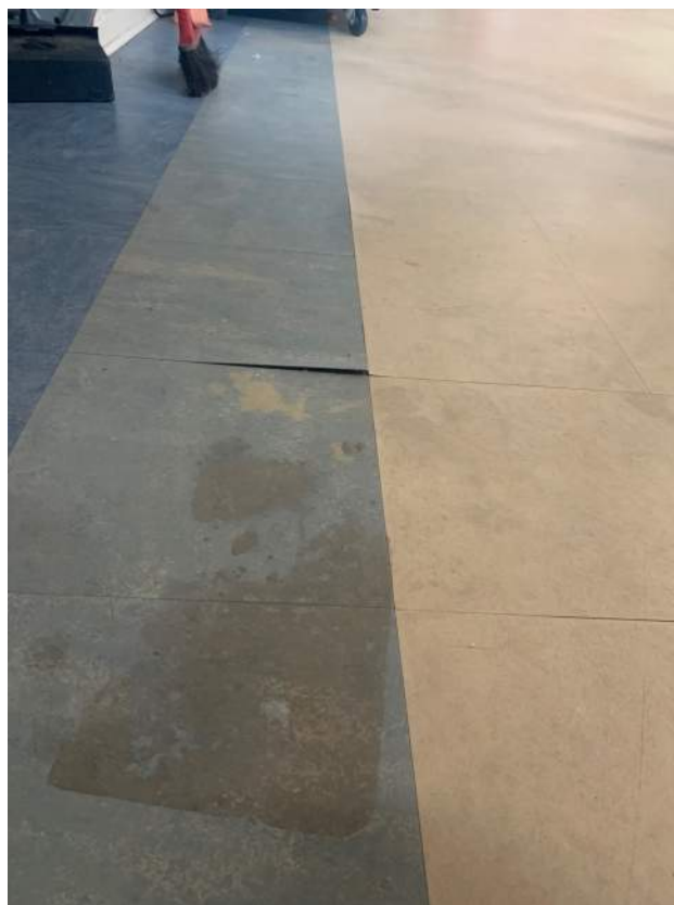
Image 2.3.6 MPR flooring. Taken on 05/02/2022 by Belli Architectural Group.
