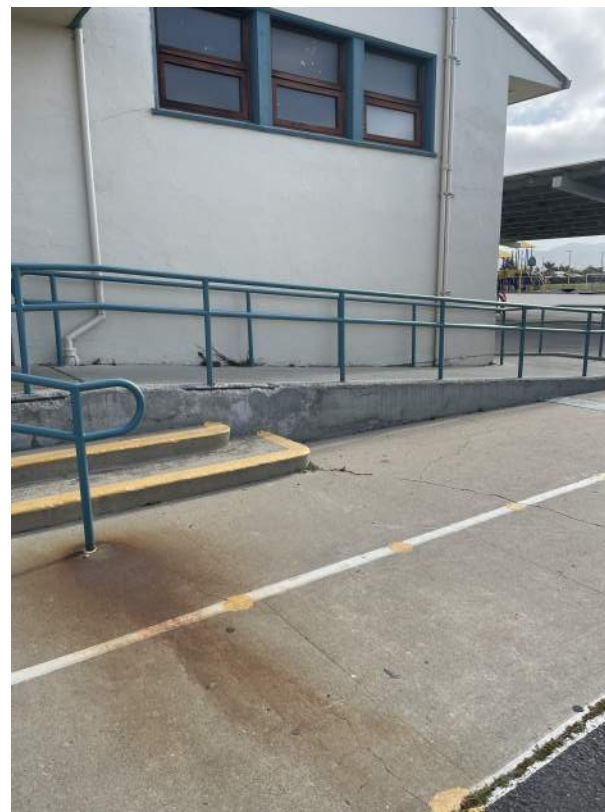
Image 2.1.2 Existing conditions at exterior pavement. Taken on 05/02/2022 by Belli Architectural Group.
