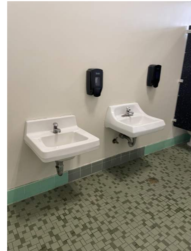
Image 2.3.3 Existing student restrooms. Taken on 05/02/2022 by Belli Architectural Group.
