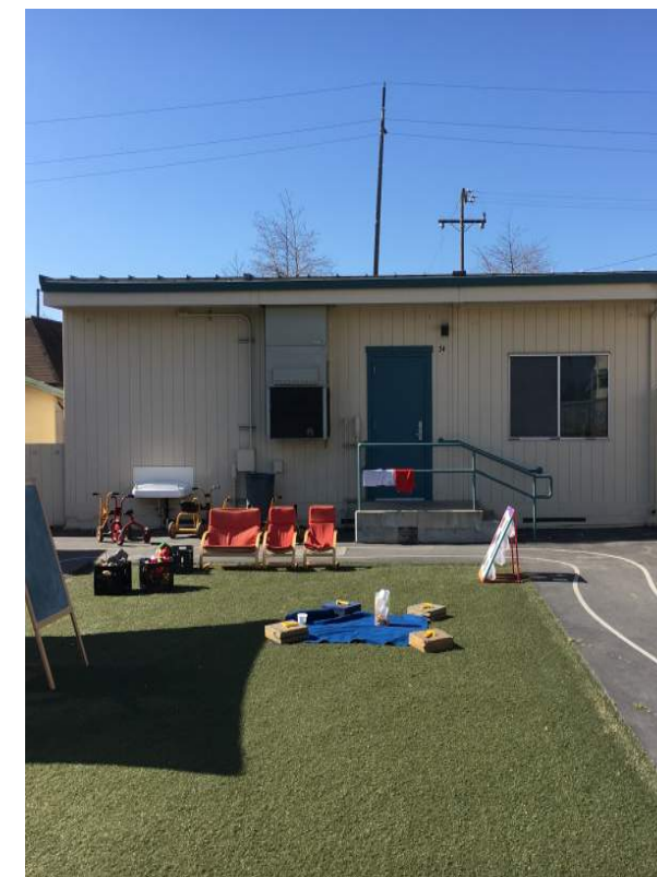
Image 2.3.10 Preschool. Non-accessible entrance. Taken on 05/02/2022 by Belli Architectural Group.
