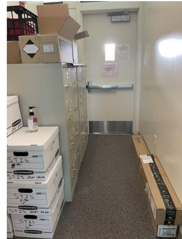
Image 2.3.4 Storage filing cabinets obstructing exit. Taken on 05/02/2022 by Belli Architectural Group.
