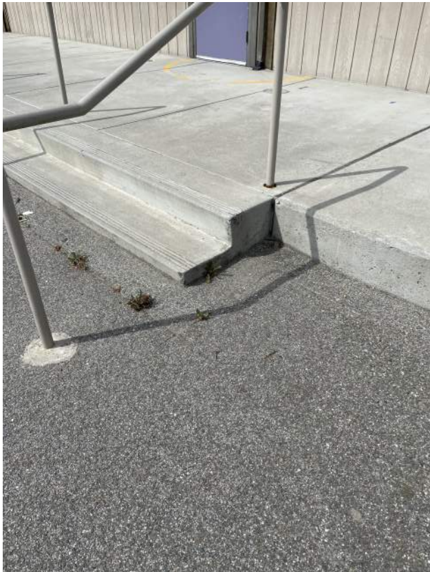
Image 2.1.2 Ingrown vegetation in asphalt. Taken on 04/26/2022 by Belli Architectural Group.
