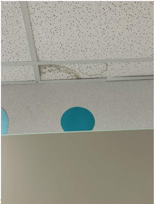
Image 2.3.3 Damaged ceiling tiles. Taken on 04/26/2022 by Belli Architectural Group.
