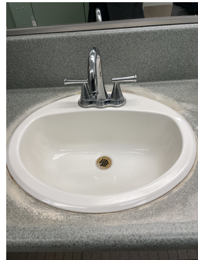
Image 2.3.1 Damaged countertop surfaces in restrooms. Taken on 04/26/2022 by Belli Architectural Group.
