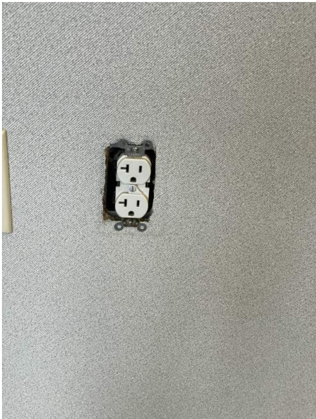
Image 2.3.2 Cover plates missing at electrical outlet. Taken on 04/26/2022 by Belli Architectural Group.
