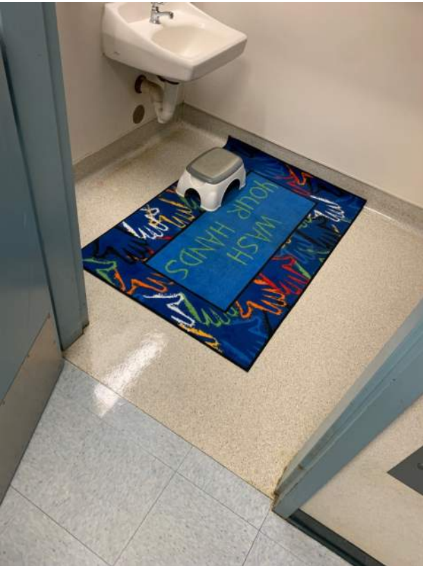
Image 2.4.1 Kindergarten/preschool sinks at non-accessible height for students. Taken on 04/26/2022 by Belli Architectural Group.
