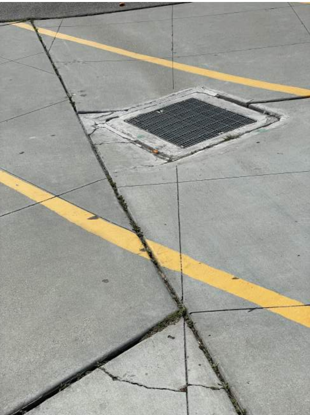
Image 2.1.1 Cracks in concrete walkways. Taken on 04/26/2022 by Belli Architectural Group.
