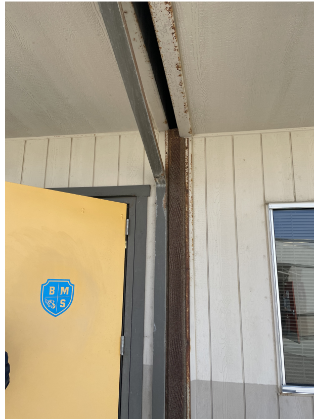
Image 2.2.2 Rust and rot at relocatable classroom. Taken on 04/26/2022 by Belli Architectural Group.
