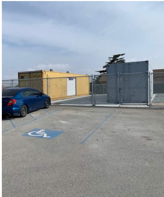
Image 2.1.6 Conex storage containers on site. Taken on 04/26/2022 by Belli Architectural Group.
