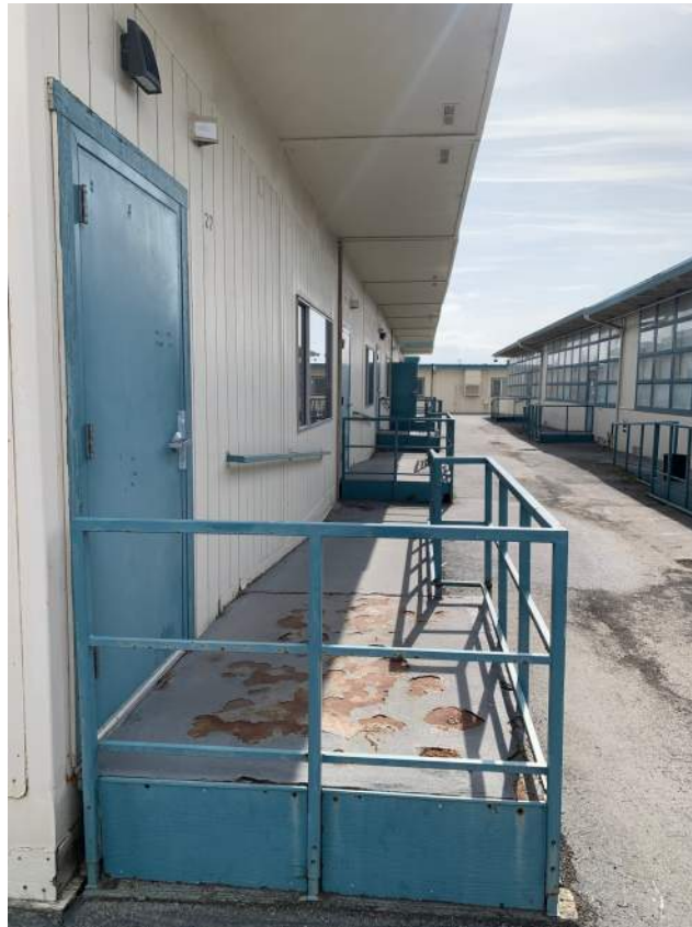
Image 2.2.4 Existing conditions at portable classrooms. Taken on 04/26/2022 by Belli Architectural Group.
