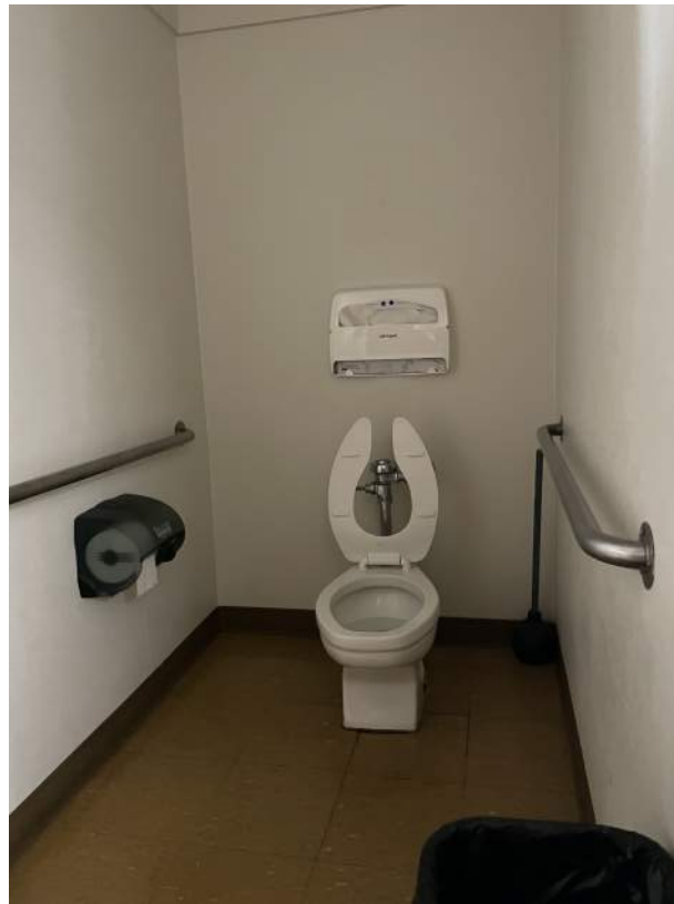
Image 2.3.7 Non-compliant restroom at Admin. Office. Taken on 04/26/2022 by Belli Architectural Group.
