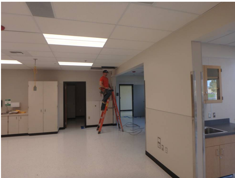
Alt. 1 main room looking southwest corner
