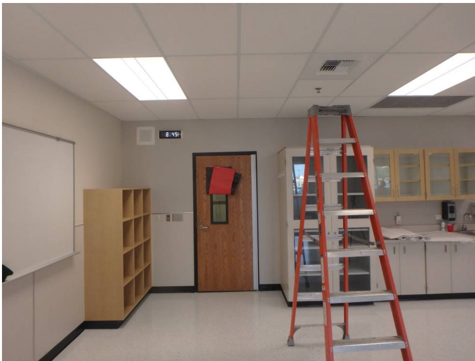
Looking at the northeast corner of the classroom and entry door
