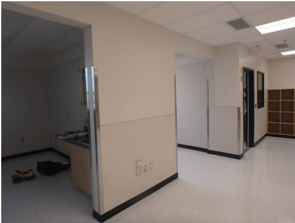
Classroom – west wall
