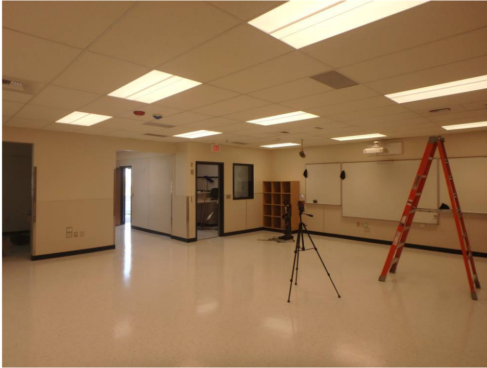
Casework in the northwest corner of the classroom
