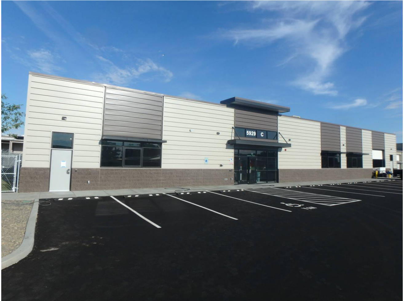
East elevation of Building Tri Tech East 1.5
