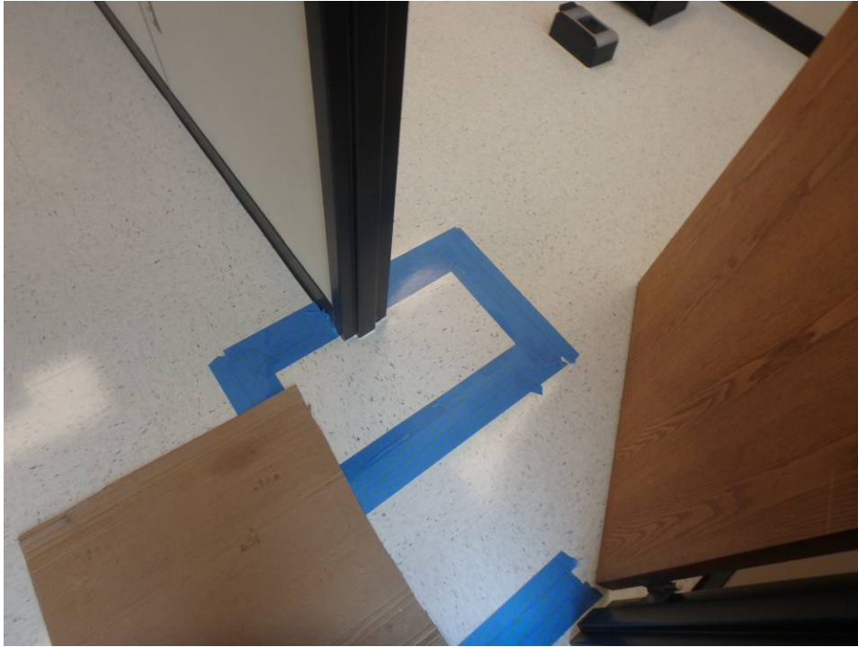
Typical repair of the VCT at the door jambs completed
