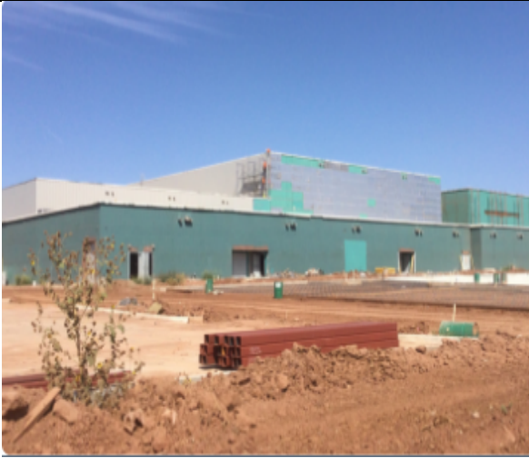
Metal Wall Panels outside Gyms
