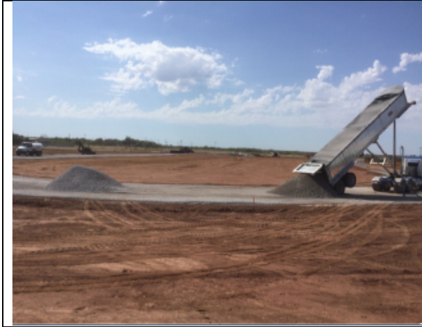
Running track rock subbase placement
