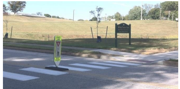
New pedestrian crosswalk installed on Red Lion Road at Valley Center Park entrance
