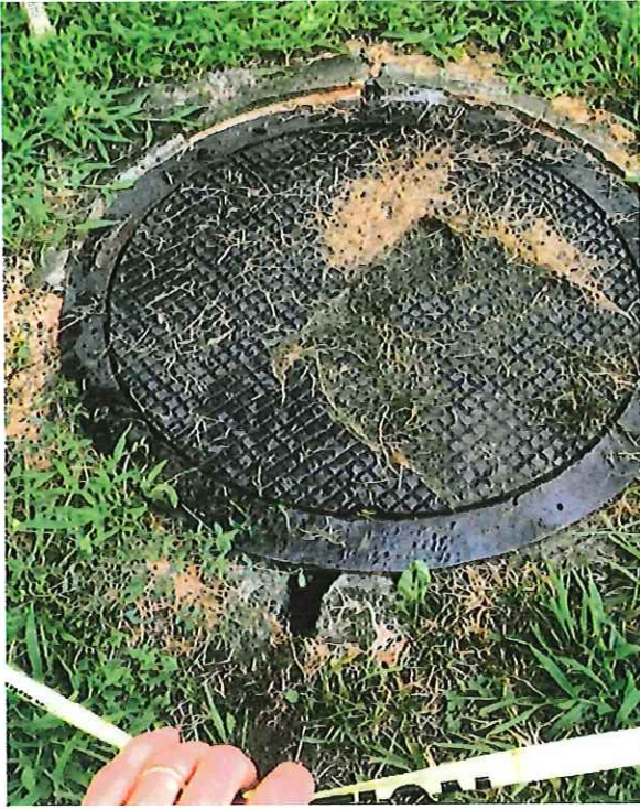
WPCA Operators fixed a manhole that was deteriorated and letting surface water into the manhole at the Suffield Middle School
