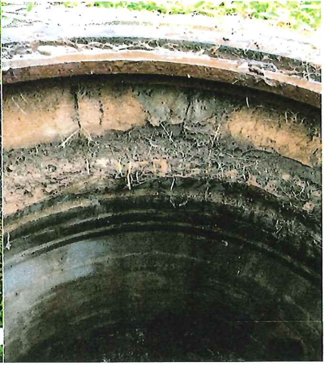
WPCA Operators fixed a manhole that was deteriorated and letting surface water into the manhole at the Suffield Middle School
