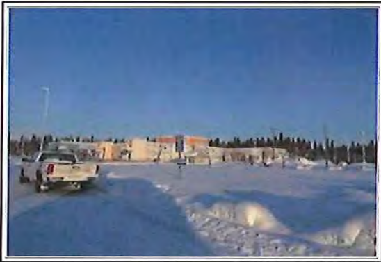
School Site Looking E Standing on Snowman Lane
