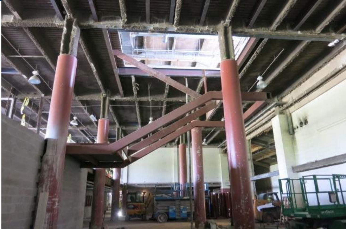
Stair C Steel being Installed
