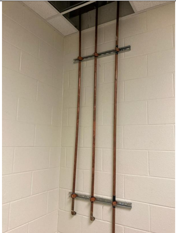
Plumbing is ongoing at custodial area.
