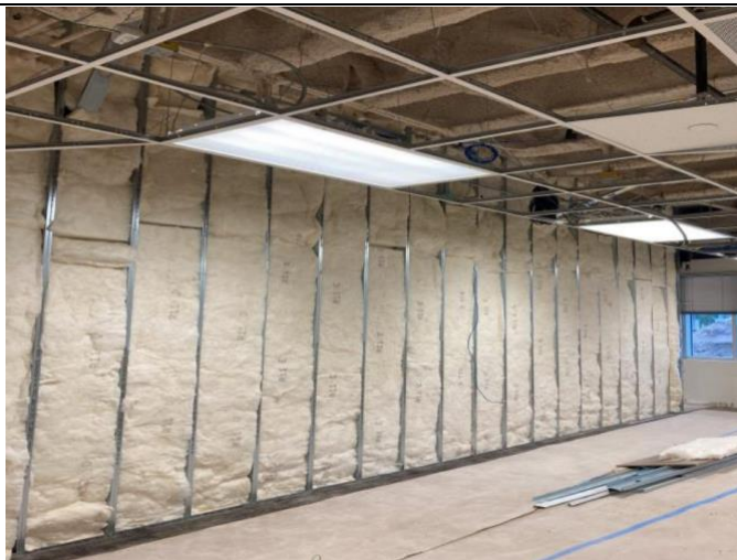
Batt insulation placement is ongoing at the temporary wall.
