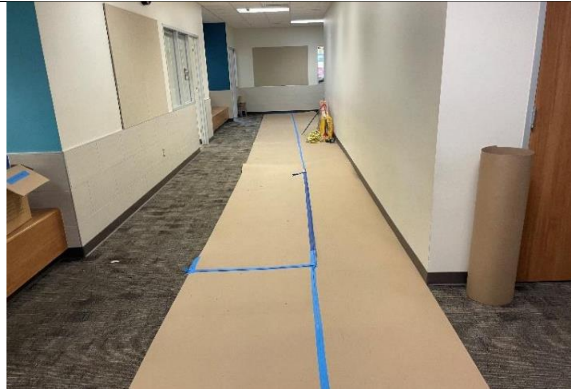
Floor protection installed for interior scope.
