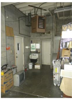
The existing heating and ventilating system is in poor condition at this time currently be used in the office space only. There is an older space heater mounted in the ceiling of the larger bay space at the old firehouse.
