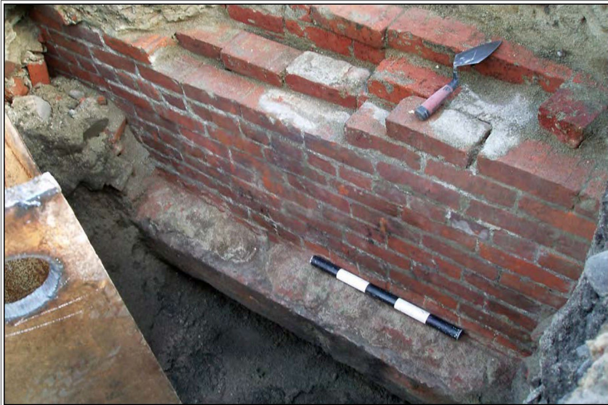
Figure 6. Example of a historic-period building foundation.
